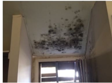
16. Historic evidence of water damage was also noted in the floor framing of the first floor bathroom. The end of one floor joist has completely rotted away and been re-supported by a 2x6 extension nailed to its end. This is not structurally sound.
