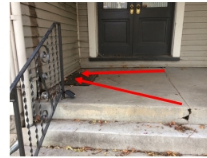
23. The home has gutters integrated into the eave framing at the edges of the roof. The eave framing and gutter on the front side of the left hand bay area is sagging away from the roof.
