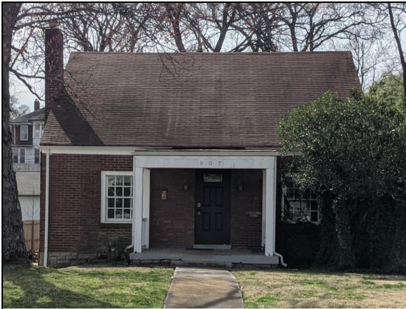
Figure 1. 907 Waldkirch Avenue, March 2021.
