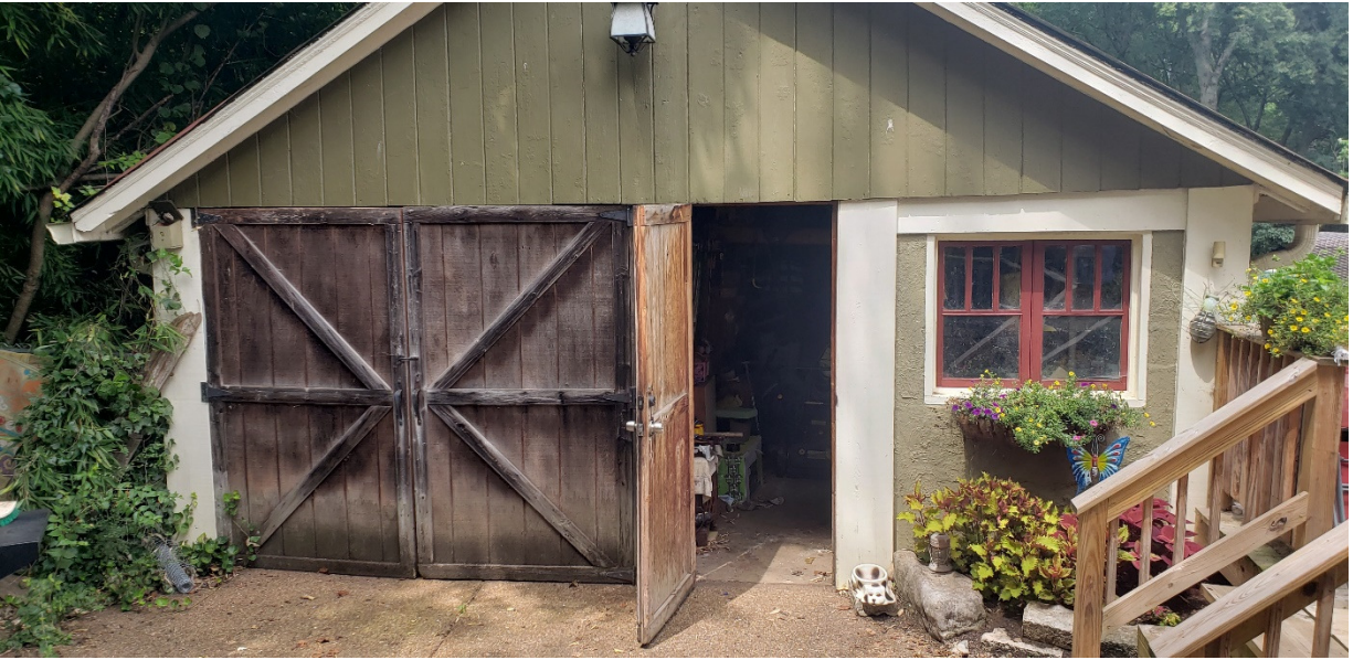
Garage/shed structure to be demolished
