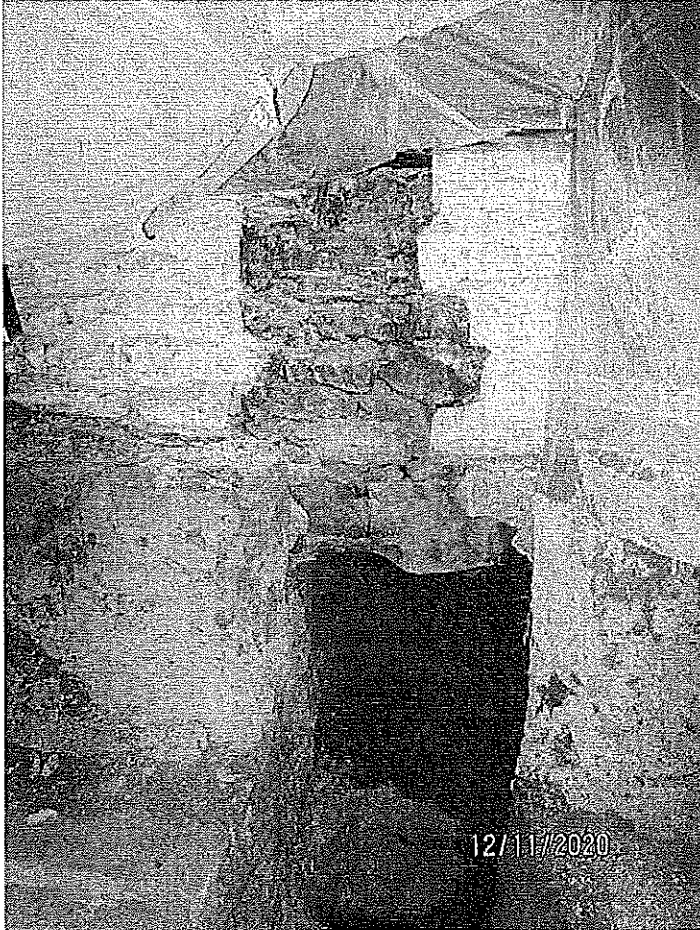
Photograph 30: Typical altered foundation wall.
