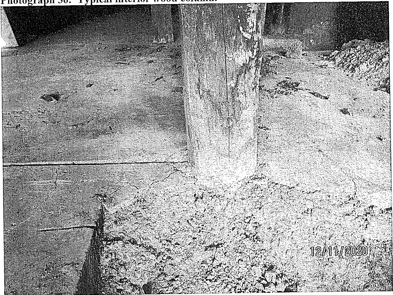
Photograph 36: Typical interior wood column.
