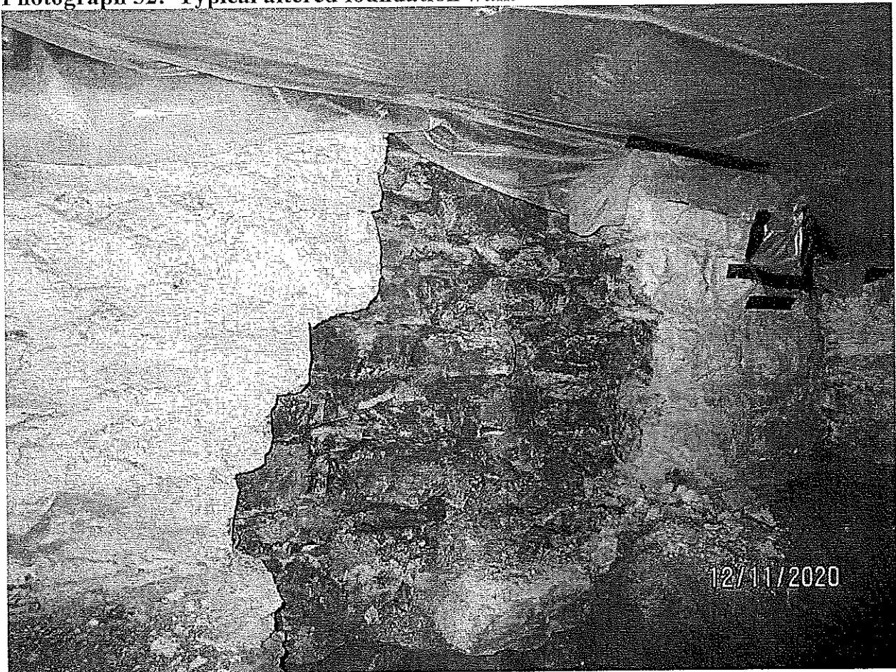
Photograph 32: Typical altered foundation wall.
