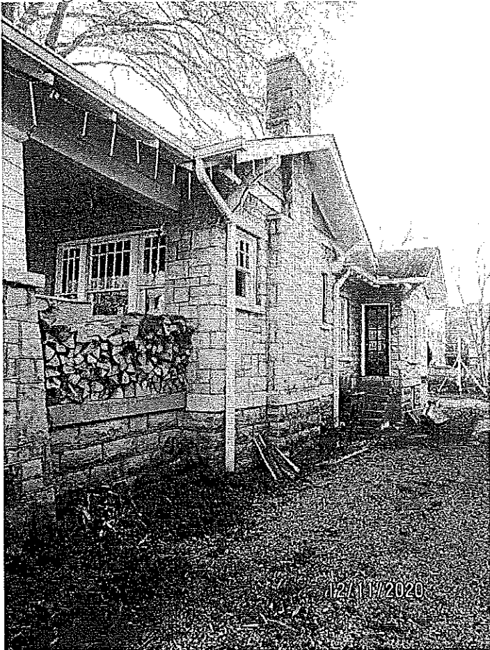
Photograph 6: Right side elevation.
