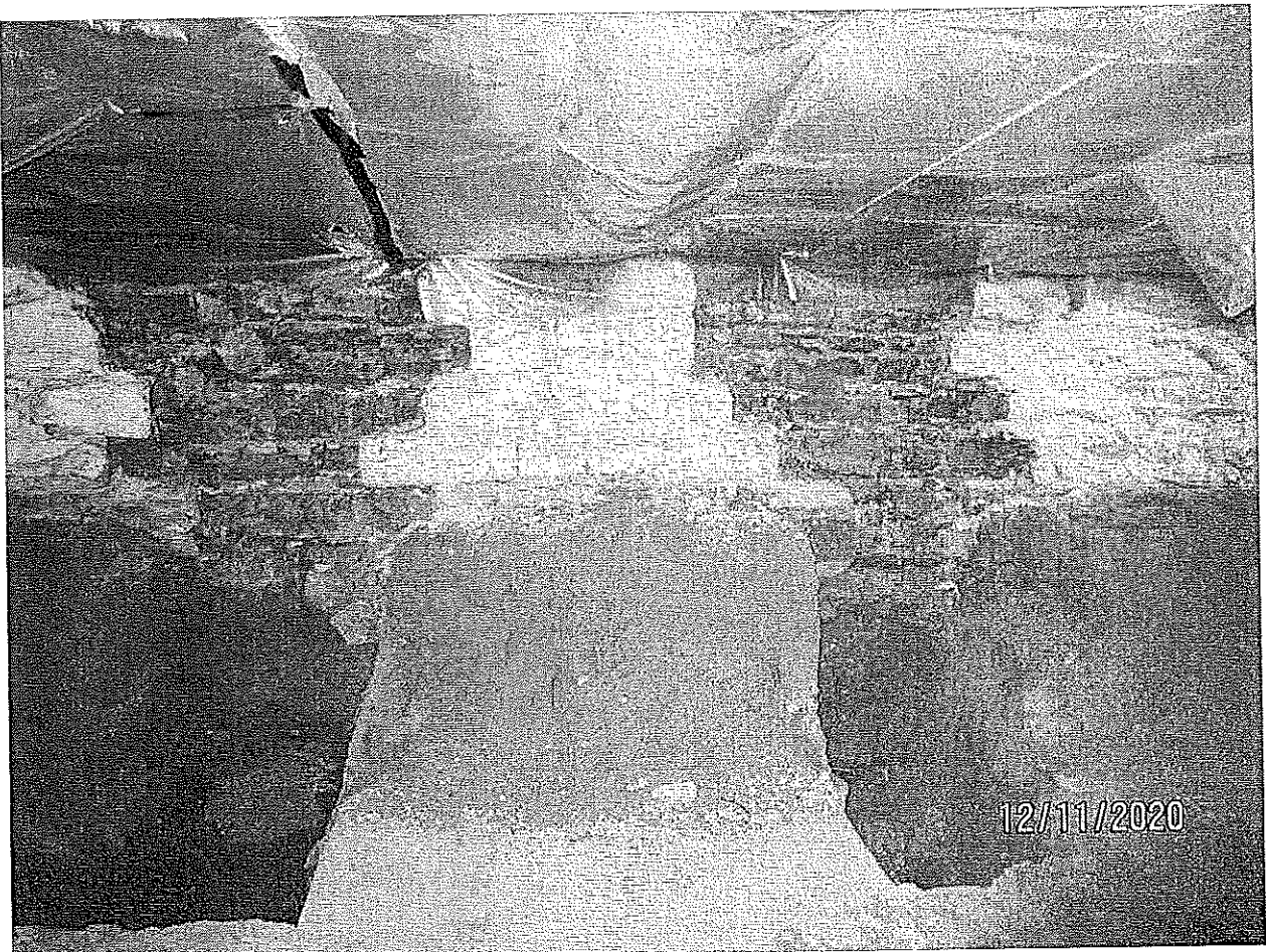
Photograph 35: Typical underpinning techniques.
