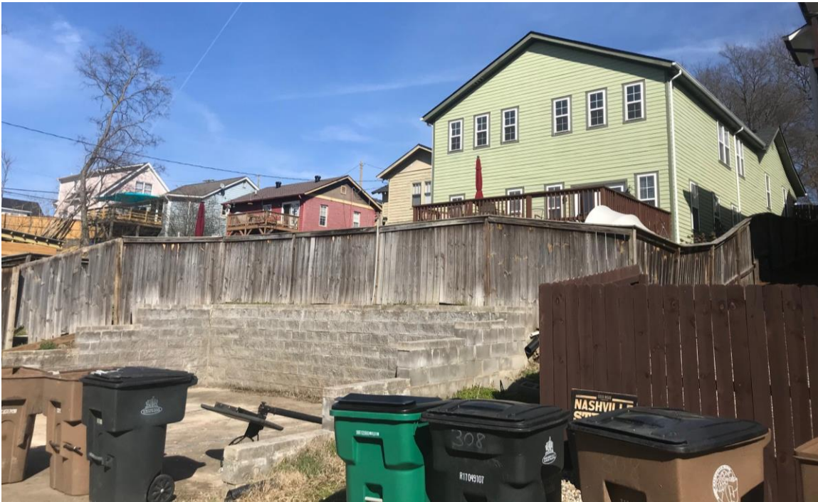
Figure 2. Area of the new garage location is limited because of the existing concrete wall.
