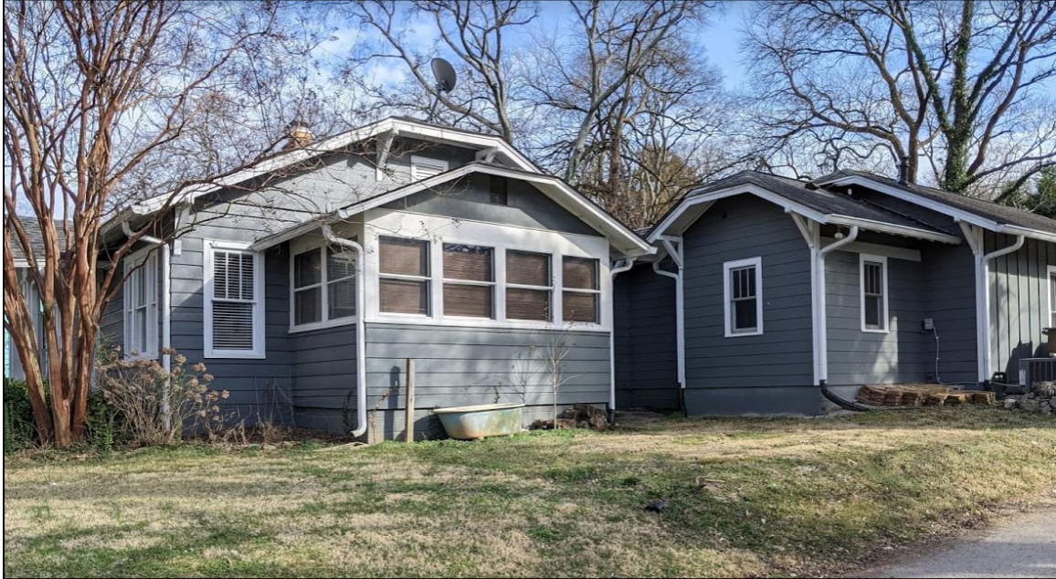
Figure 2: Existing side addition at 2529 Fairfax Avenue, and existing rear addition beyond.
