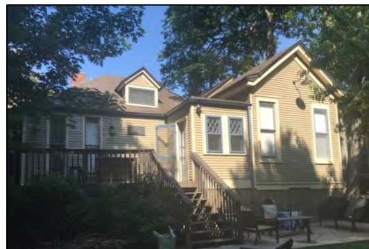
Fig. 3: Rear of 2218 Grantland Avenue, the roof of the existing addition is stepped down from the original roof.
