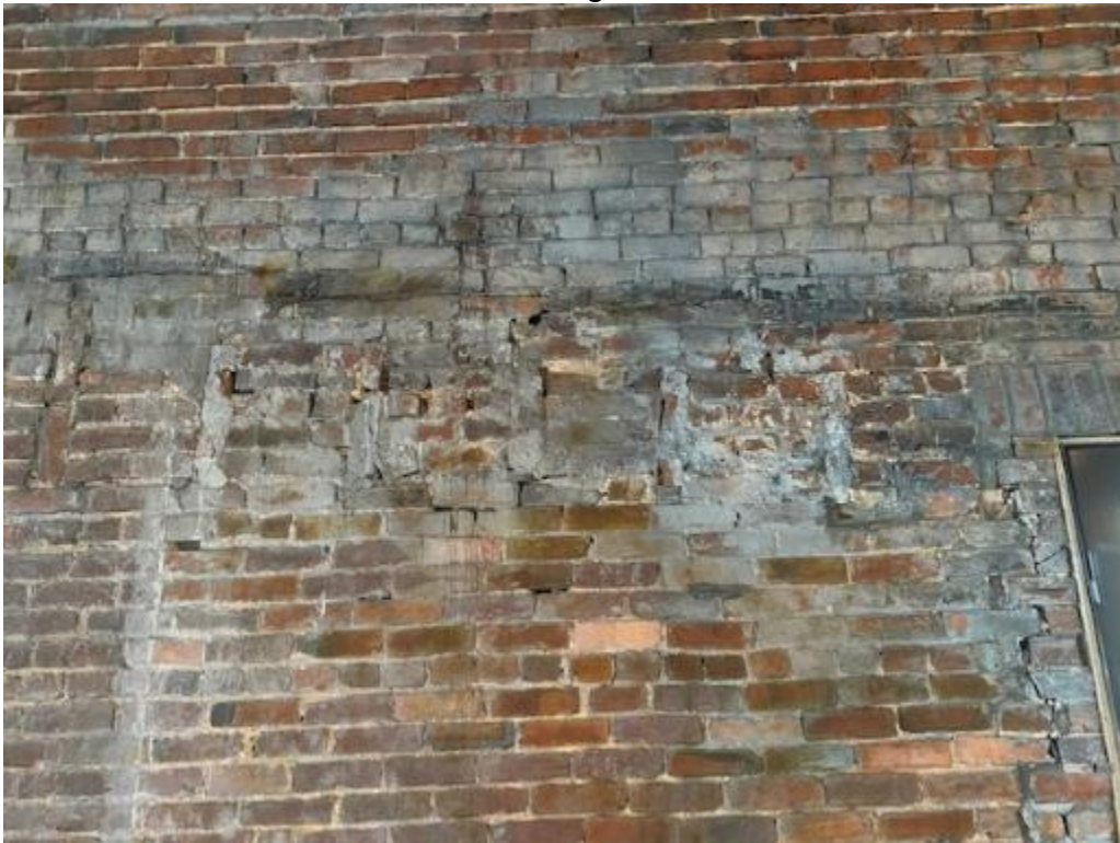
4 th floor indicating old roof line
