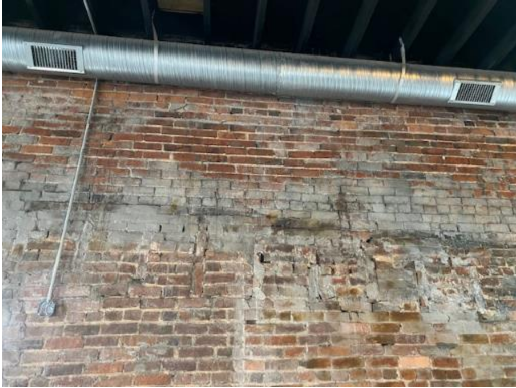
4 th floor indicating old roof line
