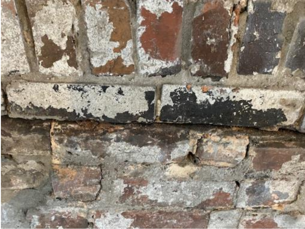
Closer view showing tar and flashing from old roof line
