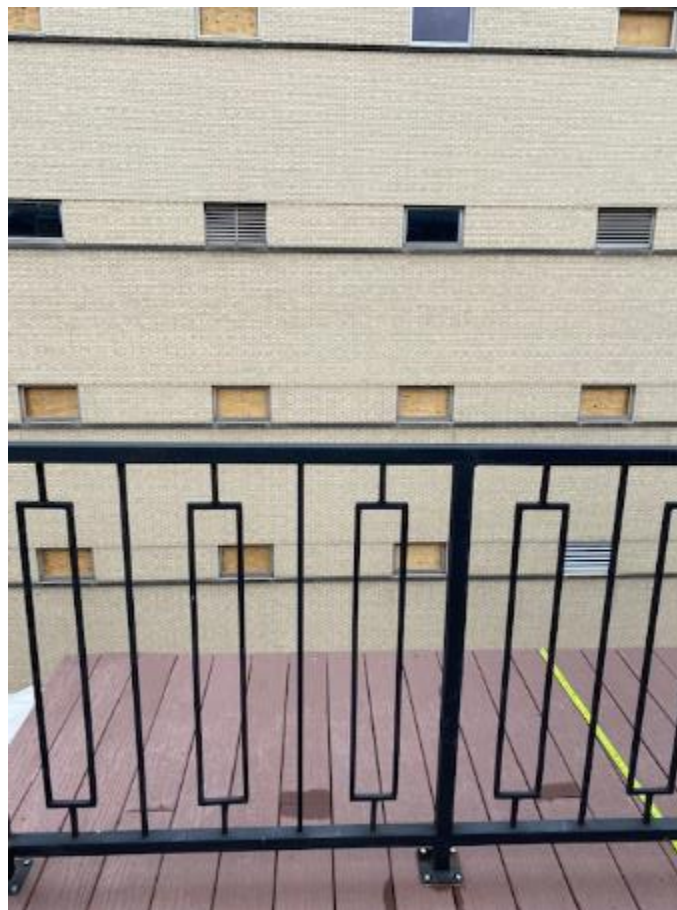
Exhibit 5 Railing and rooms with ATT building in background
