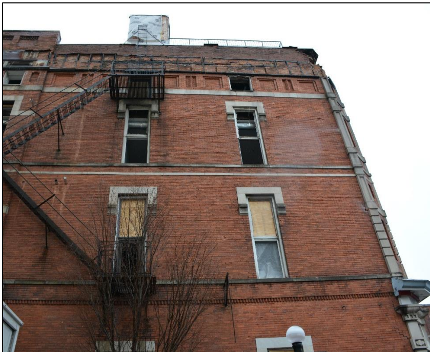
Figure 4: The railing and one of the stair towers can be seen on the Church Street side. Evidence of a missing cornice can be seen at the top of the building.
