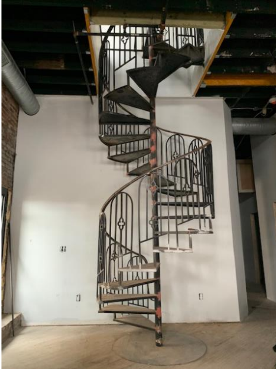
Exhibit 4 Spiral stair under the access room.
