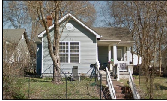
Figure 1: 1804 5 th Avenue North.
