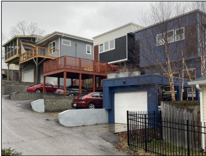
Figure 1: The rear deck at 1408 B Boscobel Street on January 25, 2021
