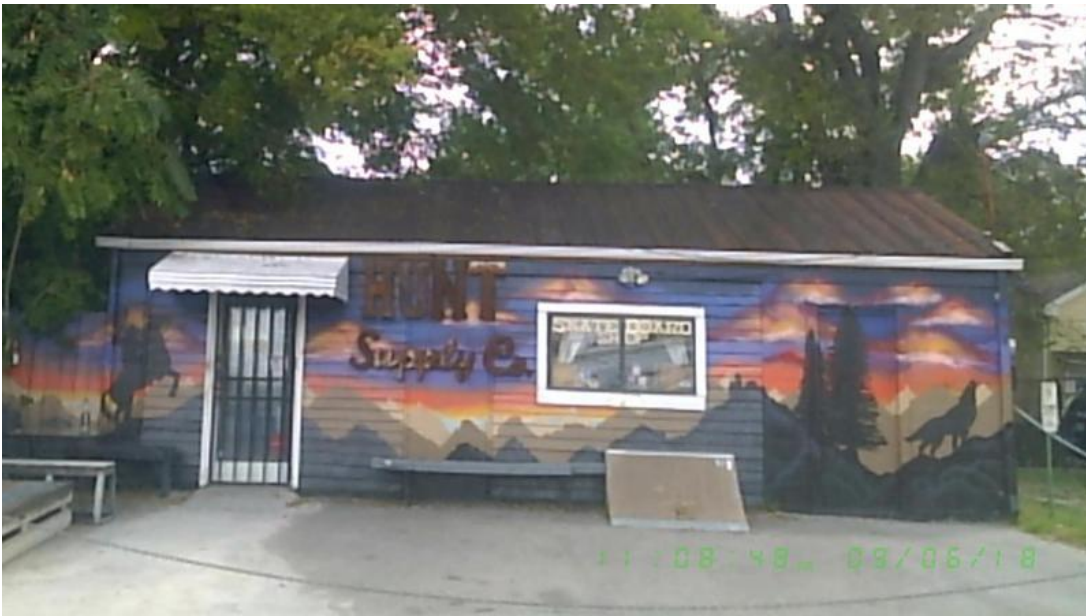
Figure 4. Rear building prior to the 2020 Tornado.
