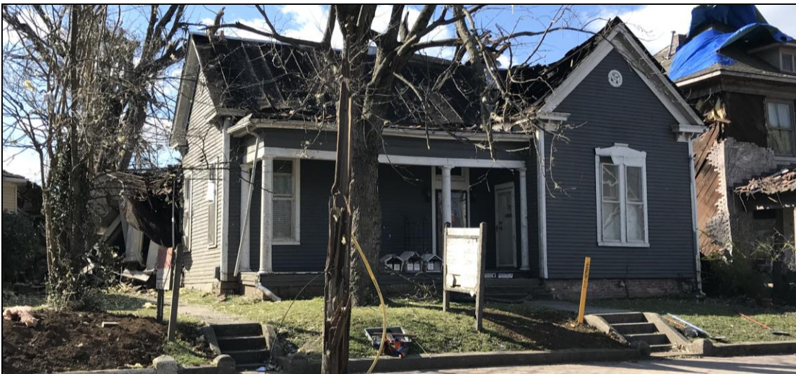
Figure 2. The tornado damage
