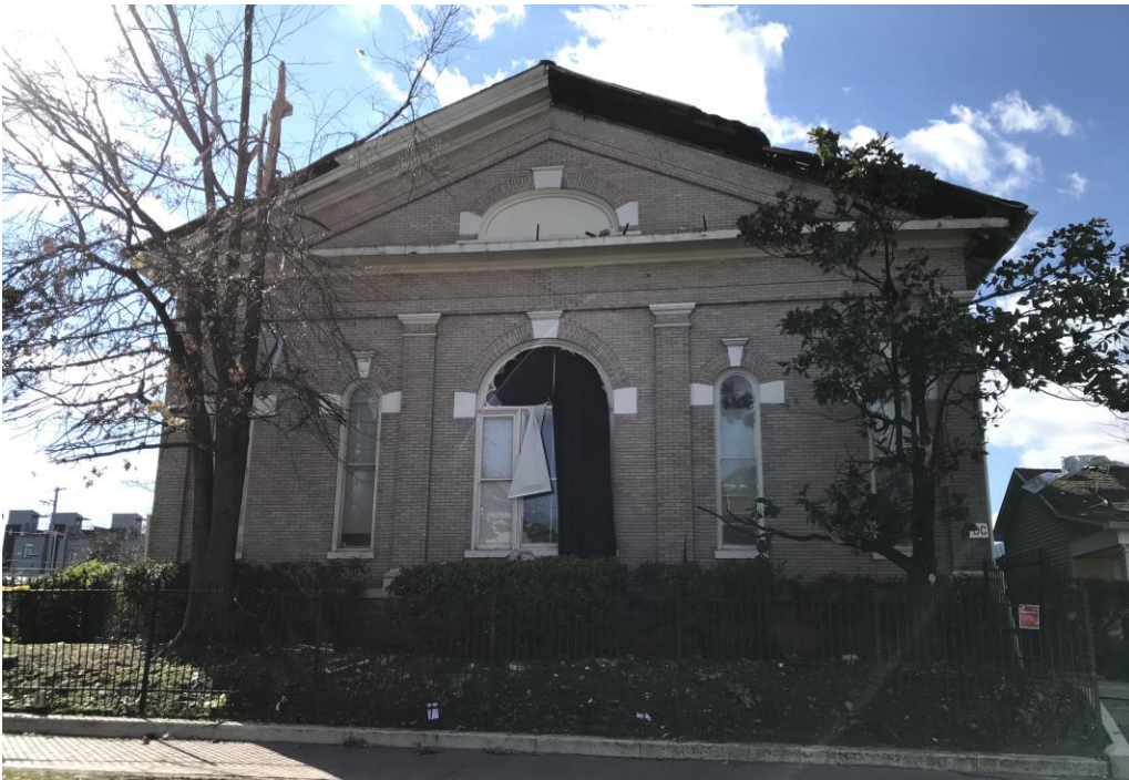
The YCAP building to the left of the site is undergoing restoration.
