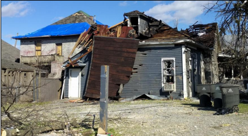
Figure 3. The tornado damage from the rear.
