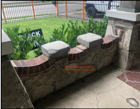
Figure 2. Center masonry enclosed porch railing.
