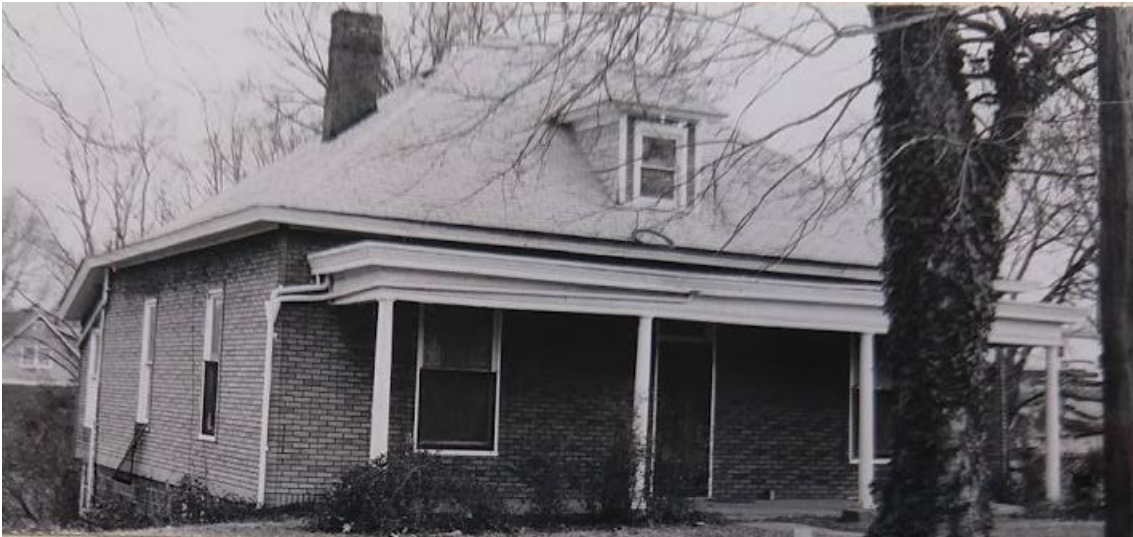
Figure 2. C. 1968 Property Assessor photo.
