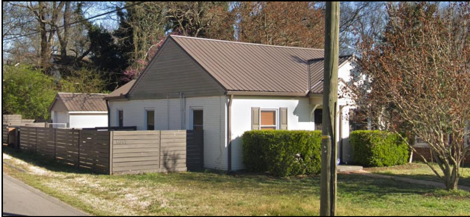
Figure 1. 1017 North 16 th Street.
