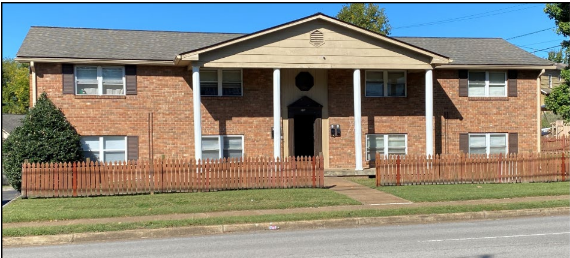
929 Boscobel, across S 10 th street, to the north
