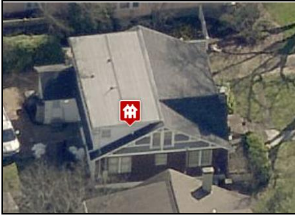
Figure 2. Rear addition and dormer to be demolished.
