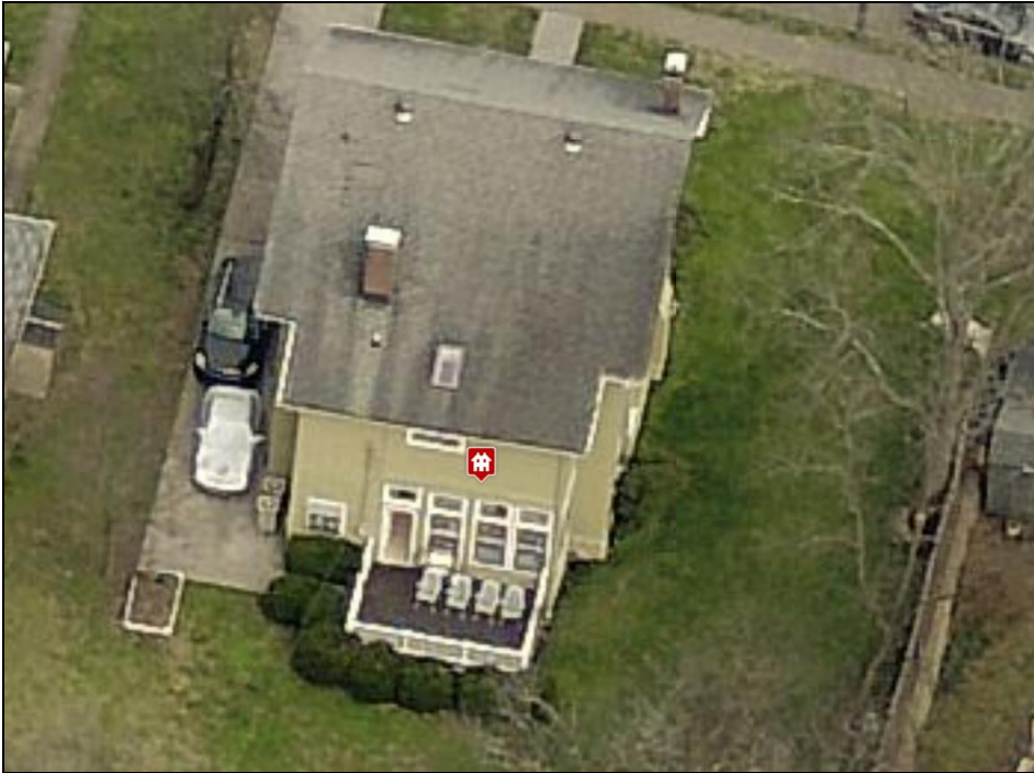
Figure 2. The two story rear addition that will be demolished.
