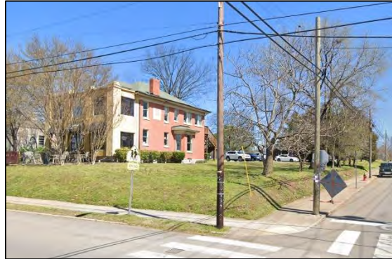
Figure 1: 201 N 11 th Street
