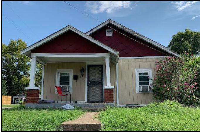
Figure 1. 1830 5 th Avenue N.
