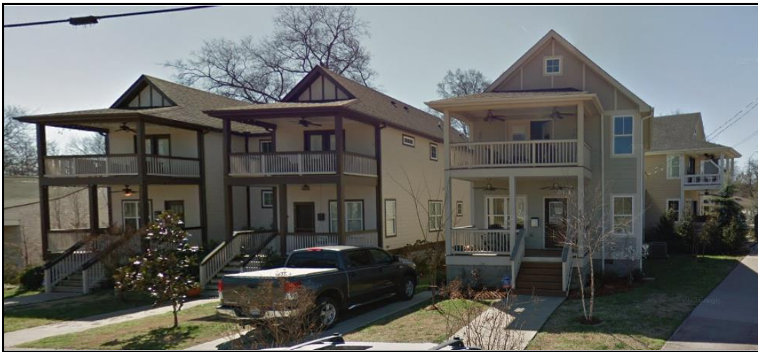
Left to right. 1829 5 th Ave N and 1831 5 th Ave N, both Non-Contributing infill approved prior to the overlay.
