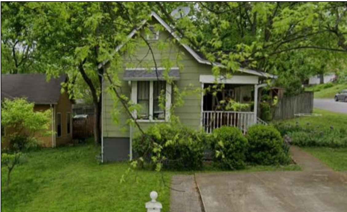
Figure 1. 1417 Russell prior to the March 3, 2020 tornado
