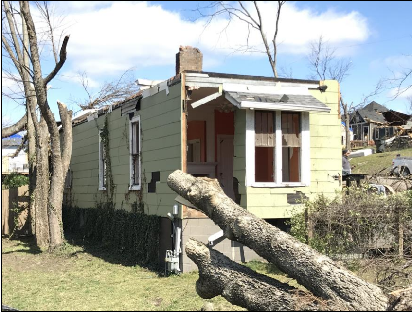
Figure 2. The tornado damage
