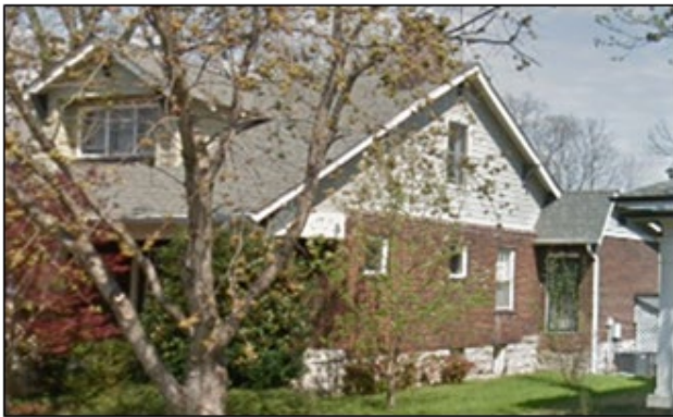
Figure 3. Right side: existing addition steps wider
