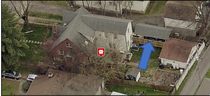
Figure 2. Carport to be demolished. The outbuilding shown near the rear property line here was demolished in December 2020.
