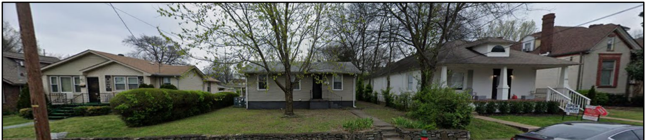
Figure 2. Streetscape. Left to right: #1012 is non-contributing, subject house, #1018 and #1020, both contributing
