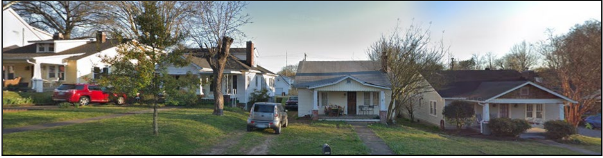
Figure 3. Streetscape. #4909, to be demolished is second from right.
