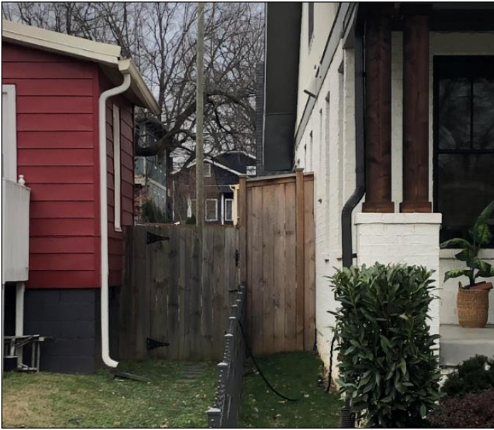
Figure 3: The fireplace is proposed on this side of the house, behind the fence.
