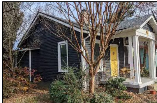
Figure 2: Left side, showing earlier addition.
