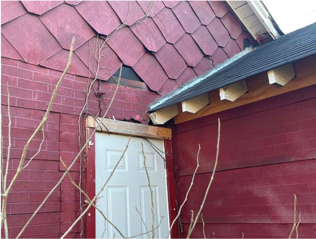
Closeup of Transition between original house and addition at the rear
