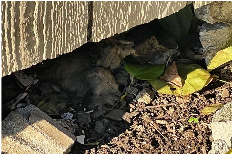
View of Crawl Space Access (9"x18")
