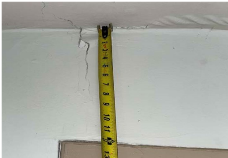
1-inch difference in door frame below
