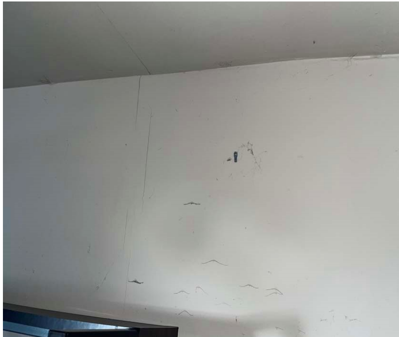
Typical cracks in drywall throughout
