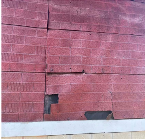
View of Damaged Siding Along South Wall
