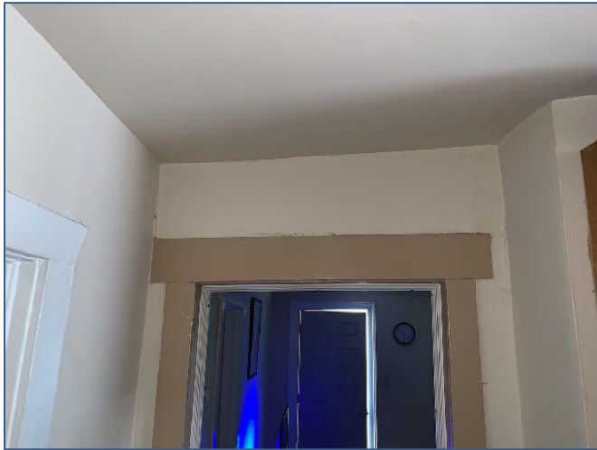
Figure 4. Sagging is evident in the interior framing.
