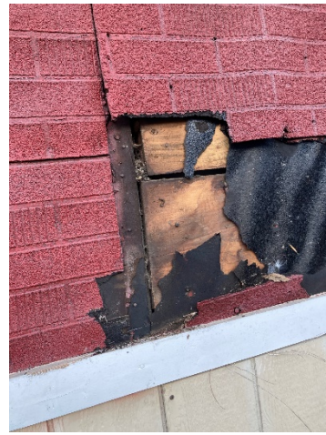
View of Damaged Siding Along South Wall
