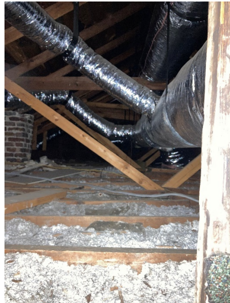
View of Rafters, Roof Framing and ceiling joists (Note diagonal and horizontal bracing)
