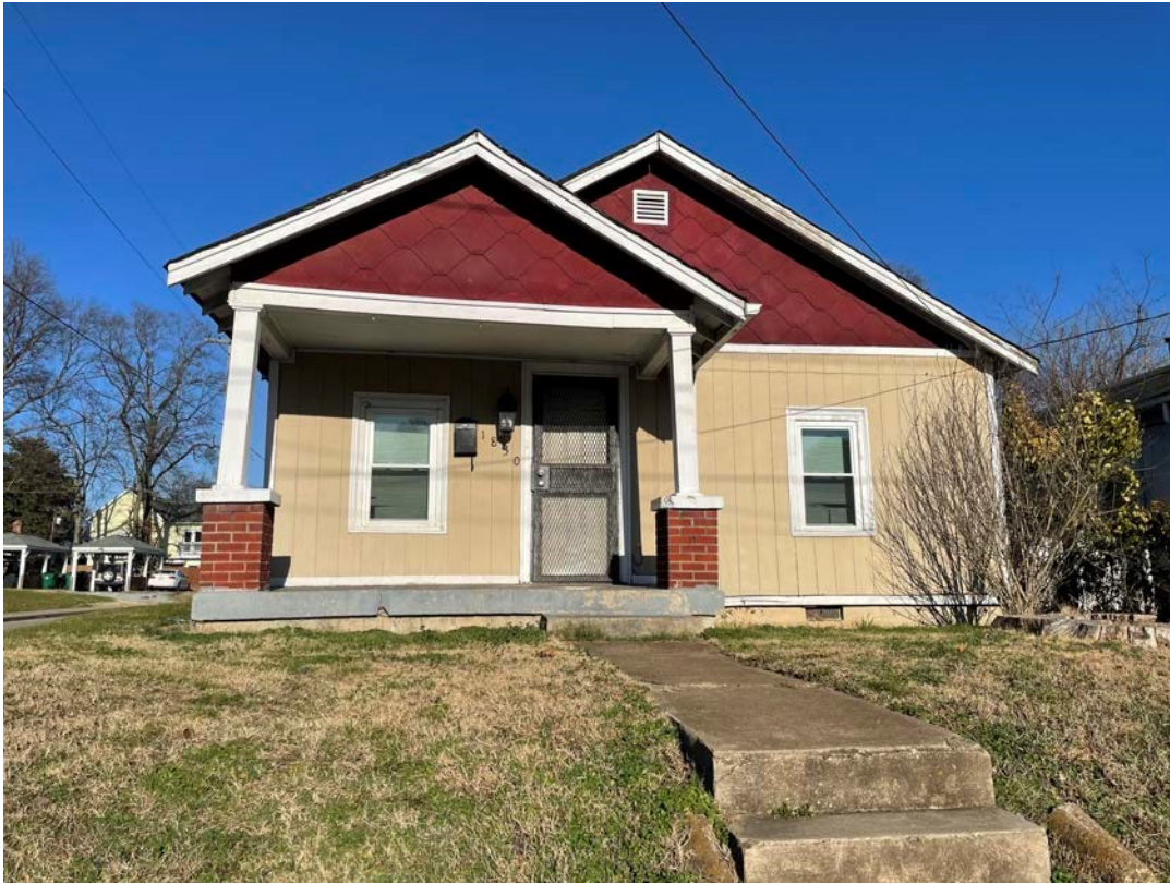
View of Front of House (Note Wood Panel Siding and Asphaltic Shingle Siding; Partial porch)
