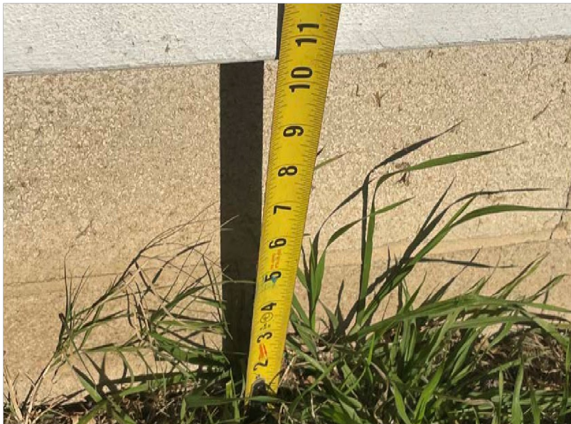
CMU Block Foundation Height less than 12"
