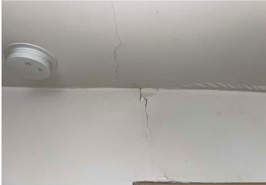
Typical cracks in drywall throughout
