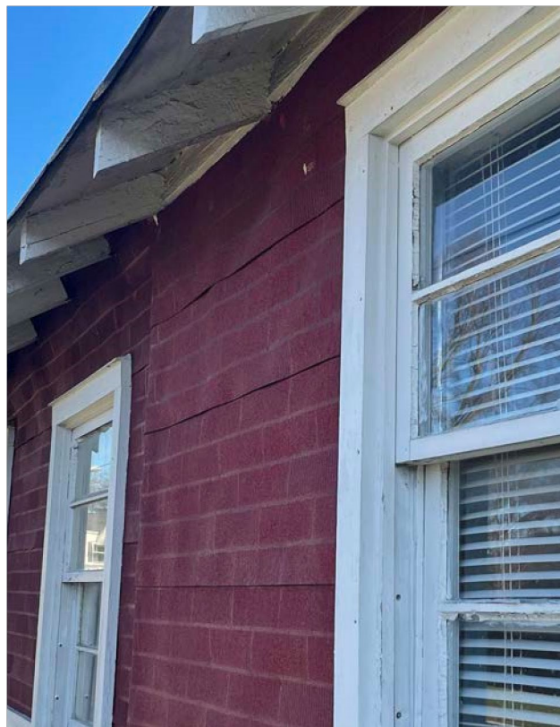
View of rafters, siding, and windows along North wall
