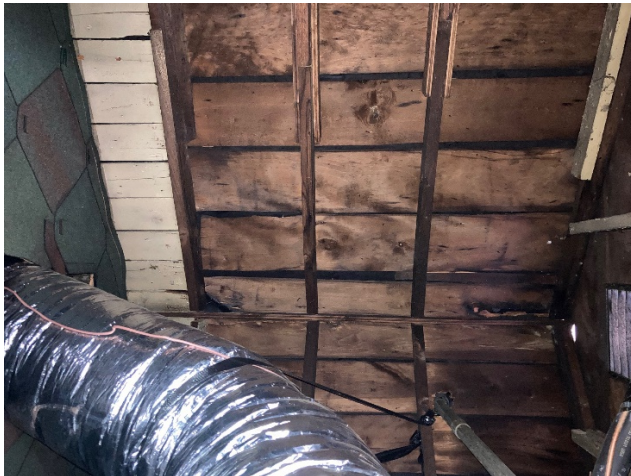
View of Rafters, Roof Framing and ceiling joists (Note diagonal and horizontal bracing)
