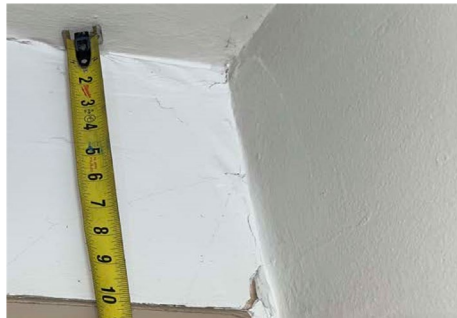
1-inch difference in door frame below
