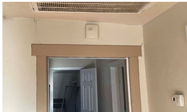
1-inch difference in door frame below
