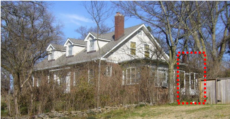
Figure 4. The area of the right façade to be removed.
