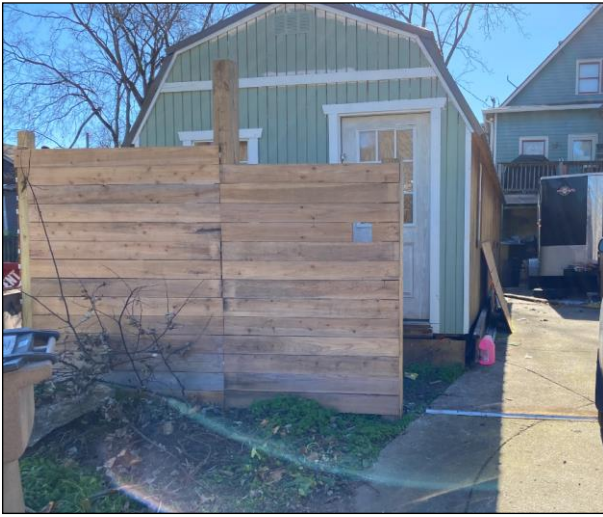
Figure 3: The outbuilding viewed from the alley.
