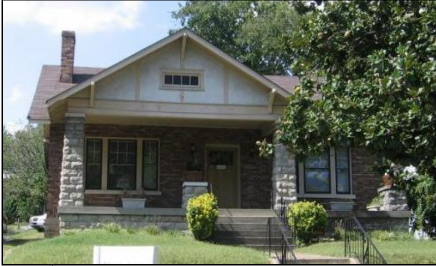
1505 16 th Avenue South – contributing; located to the right of the site
