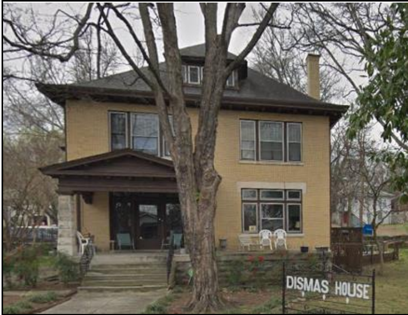
1511 16 th Avenue South – contributing; located to the immediate left of proposed in fill
