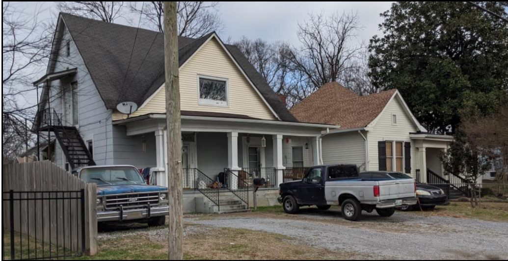
1303 and 1305 McKennie Avenue – both contributing
