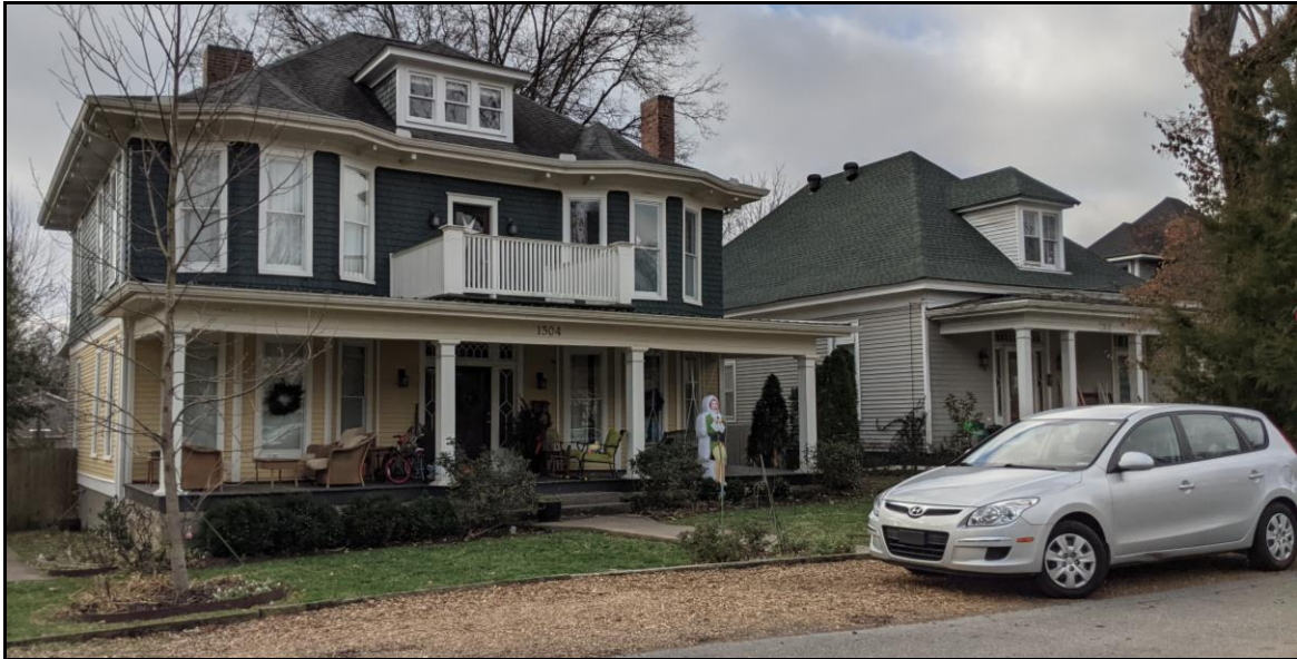
1304 and 1302 McKennie Avenue – both contributing
