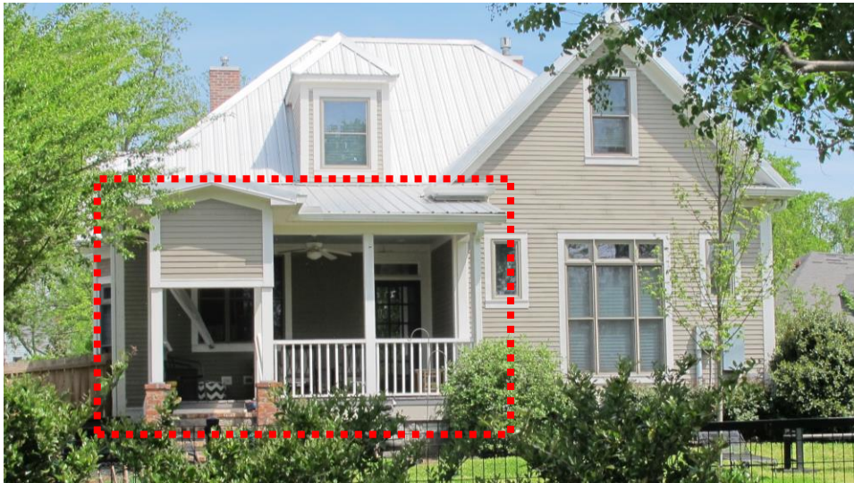
Figure 4 shows the area of demolition at the rear of the building.
