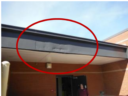
PHOTO #3: Glenview Elementary School Damaged exterior building side roof surface
