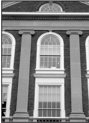
When window replacement is appropriate, they should match the originals.
