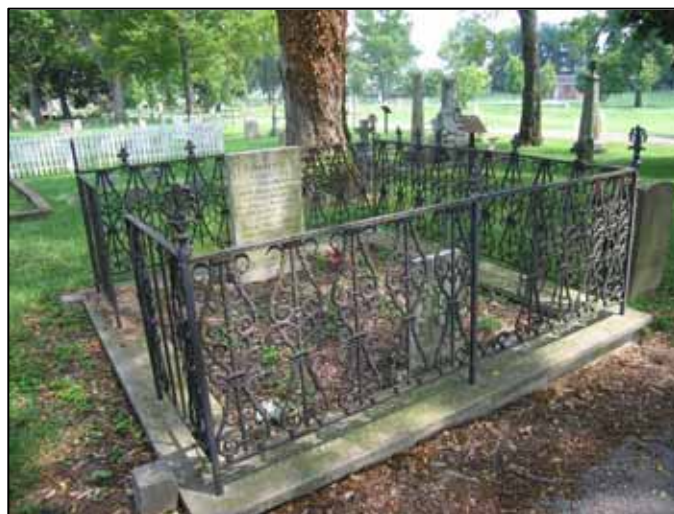
The gravesite of the daughter of William Robertson has been impacted by vandalism and theft. The ornate iron fence's gate is missing and one of the ornate cast iron panels has been stolen.
