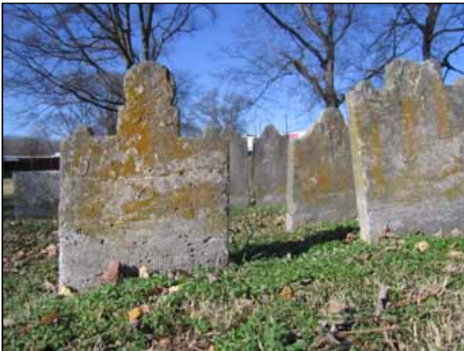
Many marble and Tennessee limestone markers are eroding
