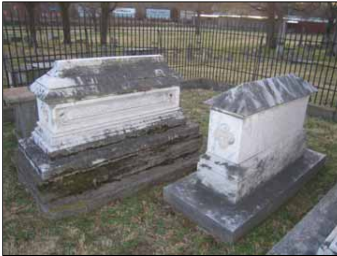
Repair work needs site-by-site and stone-by-stone attention to detail
