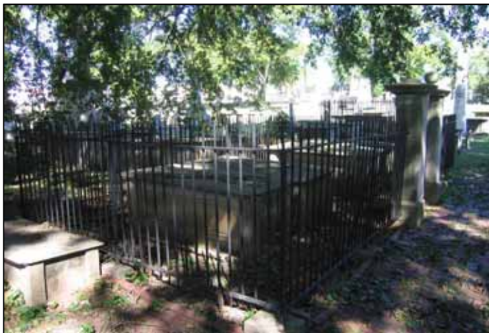
Above 2 photos: Robertson Family plot is a good example for a future demonstration restoration.
