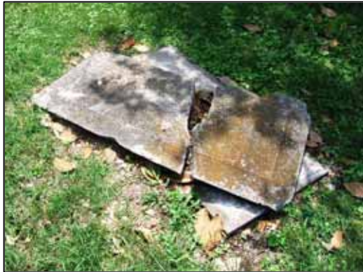
Ground tablet appears to have been impacted by a mower deck and pushed off its base.
