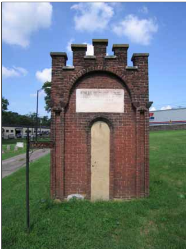
Mausoleums are in need of stabilization, similar to small building restoration
