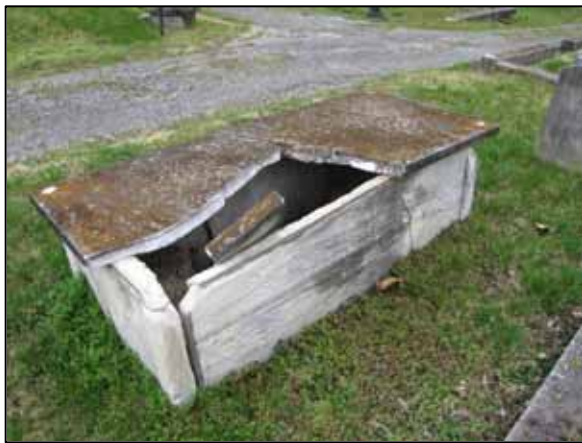
Numerous box tombs throughout cemetery are in dire need of repair
