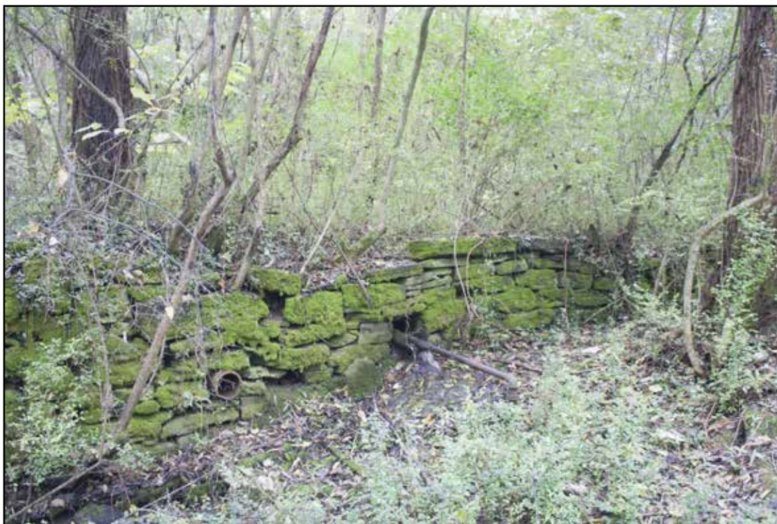
Figure 4.9. Lower retainer wall/possible Structure 11 foundation.
