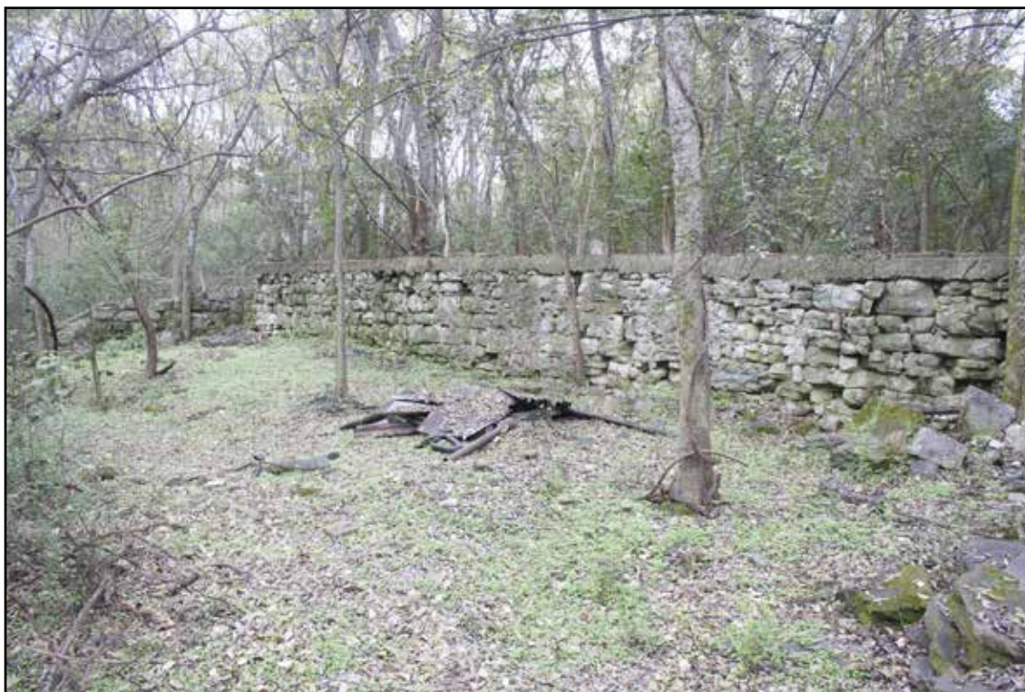
Figure 4.13. Structure 12 retainer wall/foundation.
