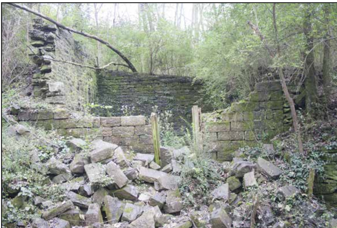
Figure 4.8. Spring house (Structure 10).
