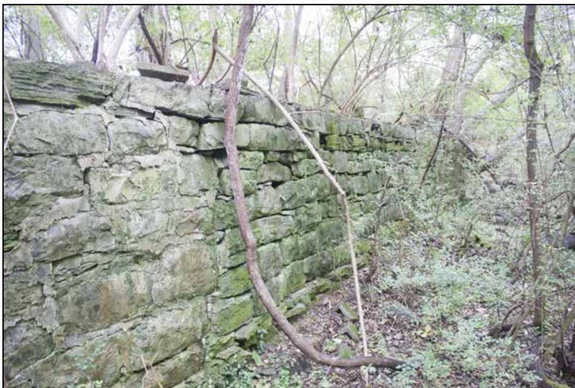
Figure 4.14. Dairy Barn (Structure 13) foundation.
