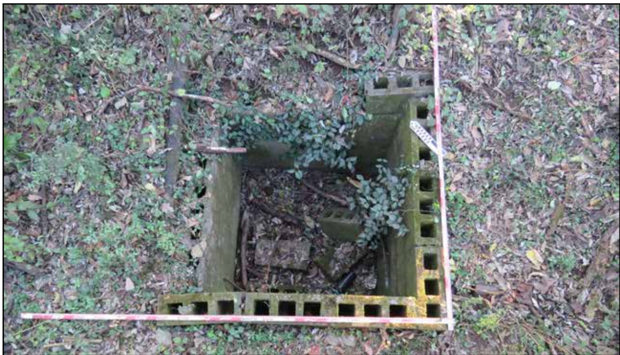
Figure 5.21. Concrete block cistern.
