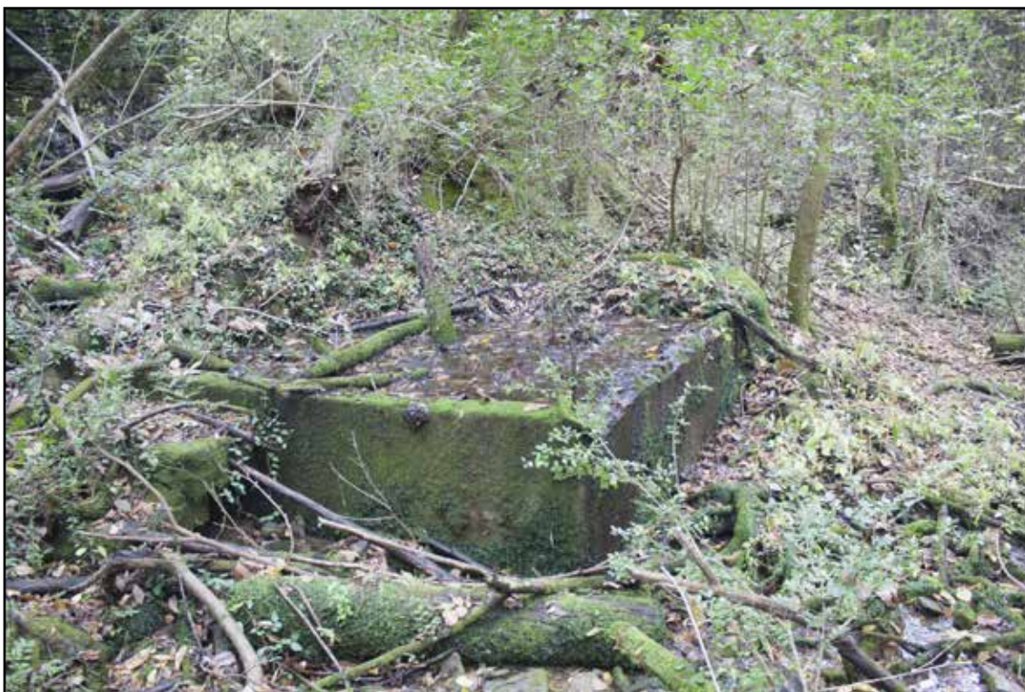
Figure 4.12. McGavock Springs (Structure 14) concrete spring house.
