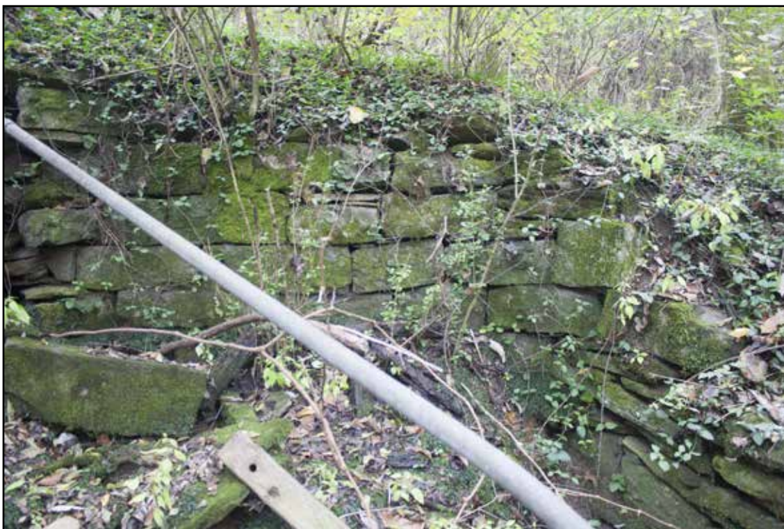
Figure 4.11. McGavock Springs (Structure 14) stone spring house.
