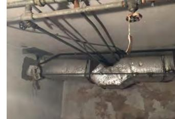
Galvanized domestic water pipes run throughout the basement
