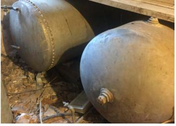
Water tanks in Room 007 once provided steam heat for the radiator system
