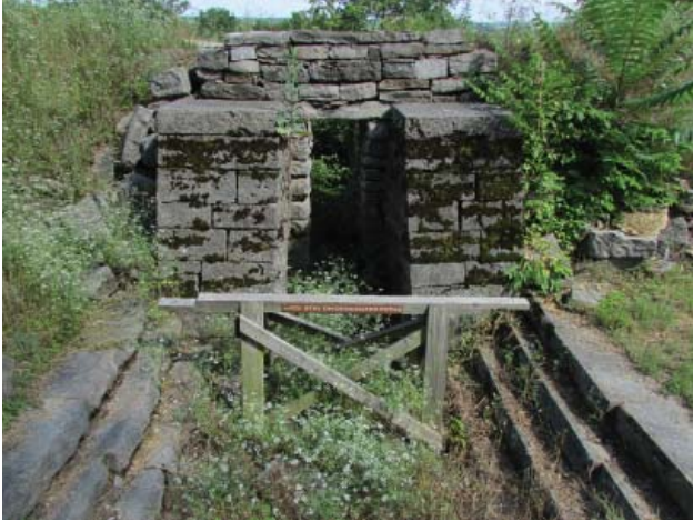
Figure 18 (above). East Bastion Tunnel (JMA, 2013).
