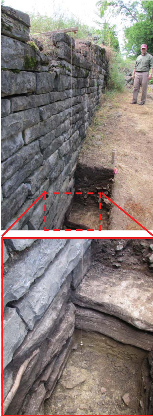
Figure 64. Wall conditions above and below grade at Test Pit 2 (1200AE, 2013).
