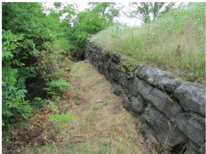
Figure 73. Typical sloped grades at top and bottom of redan walls (1200AE, 2013).
