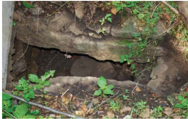
Figure 41. Drop inlet, cover removed (JMA, 2013).
