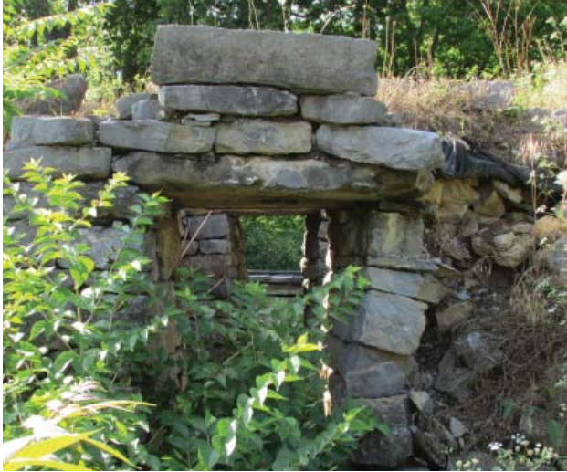
Figure 89 (above). East Bastion tunnel (east end) with partial collapse and instability in masonry above (1200 AE, 2013).
