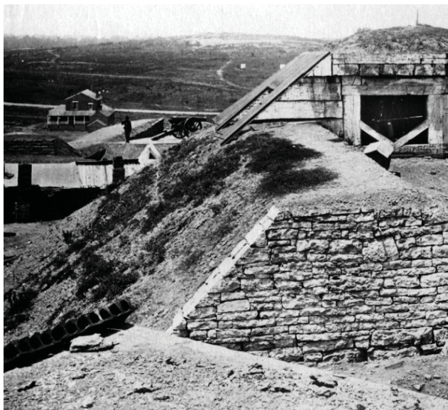
Figure 11. 1864 photograph at South Sally Port and bombproofed Casemate No. 1. Coursed rubble exterior stone facing with rough rock-faced texture. Library of Congress (FNVC).
