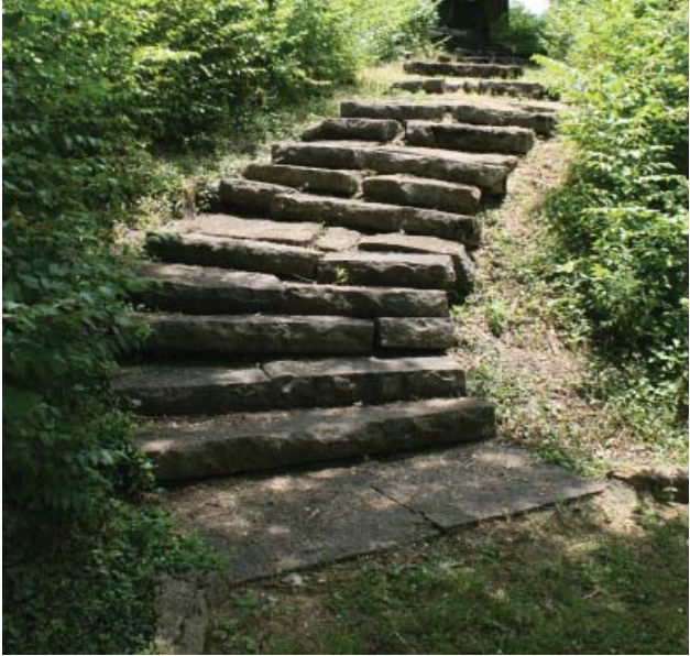
Figure 44. Limestone slab stairway leads up hill to fort structure (JMA, 2013).
