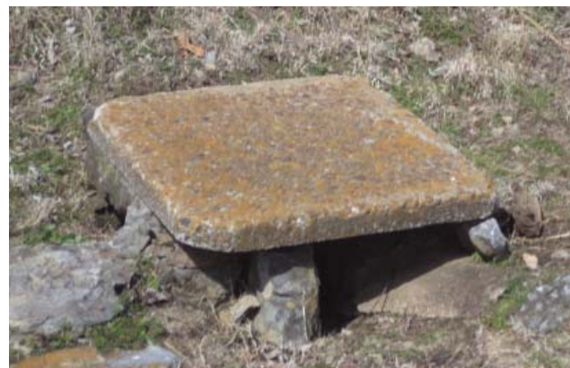
Figure 43. Concrete replacement cap for inlet set on stone corner blocks (JMA, 2013).
