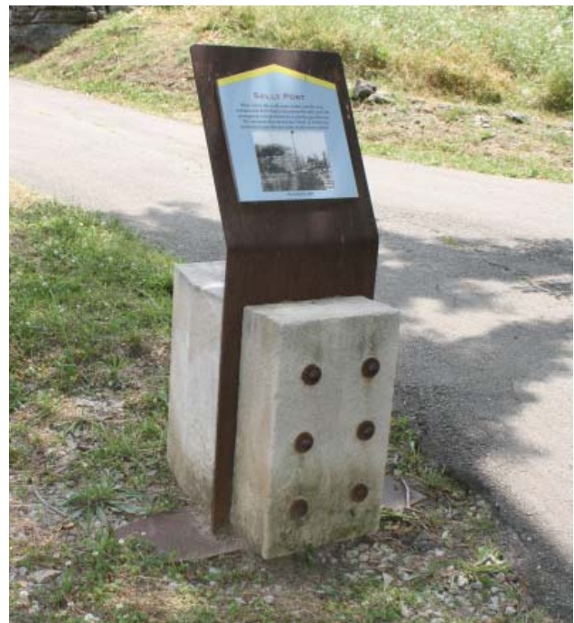
Figure 53. Steel plate with interpretive sign sandwiched between and through-bolted to plinth blocks, installed 2004 (JMA, 2013).
