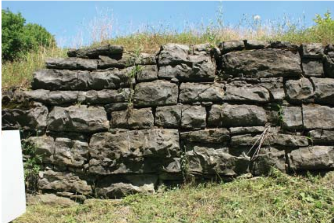
Figure 15. Coursed rough dry-stacked masonry (JMA, 2013).
