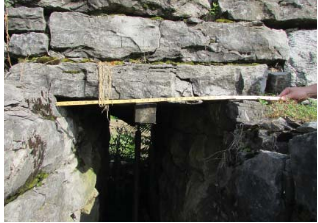
Figure 89 (above). East Bastion tunnel (east end) with partial collapse and instability in masonry above (1200 AE, 2013).
