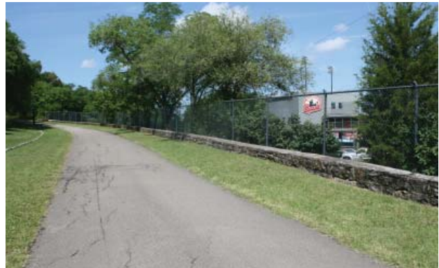
Figure 30. Low stone retaining wall parapet along the south side of loop road (JMA, 2013).
