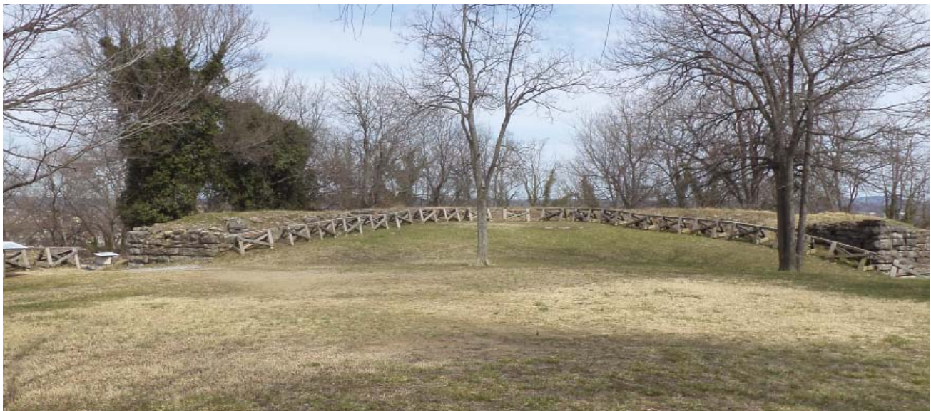
Figure 56 (below). Barricades installed 2004 (JMA, 2013).
