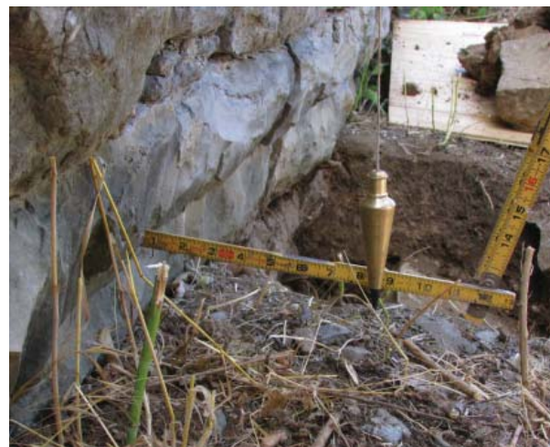
Figures 58a and 58b. Wall profile survey method with masons rule and plumb-bob (plummet) at horizontal joints at top, middle, and bottom of wall (1200AE, 2013).
