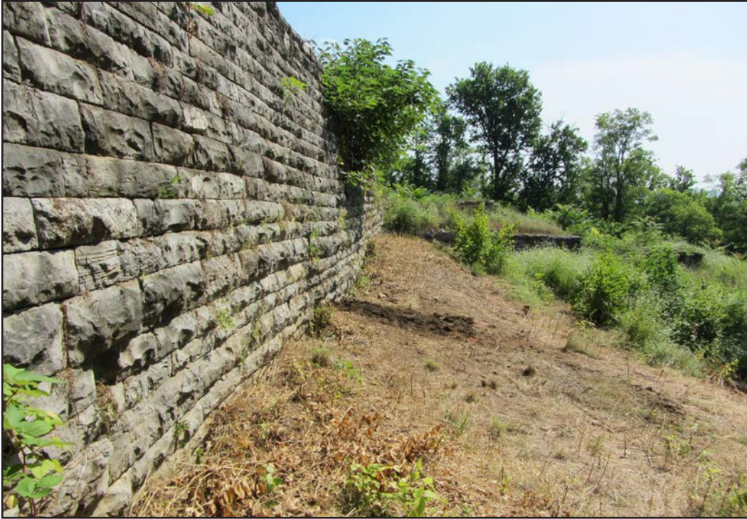
A. Location of Trench 1, Facing East along the South Wall
