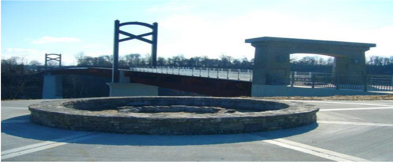
Cumberland River Pedestrian Bridge – Stones River Greenway
