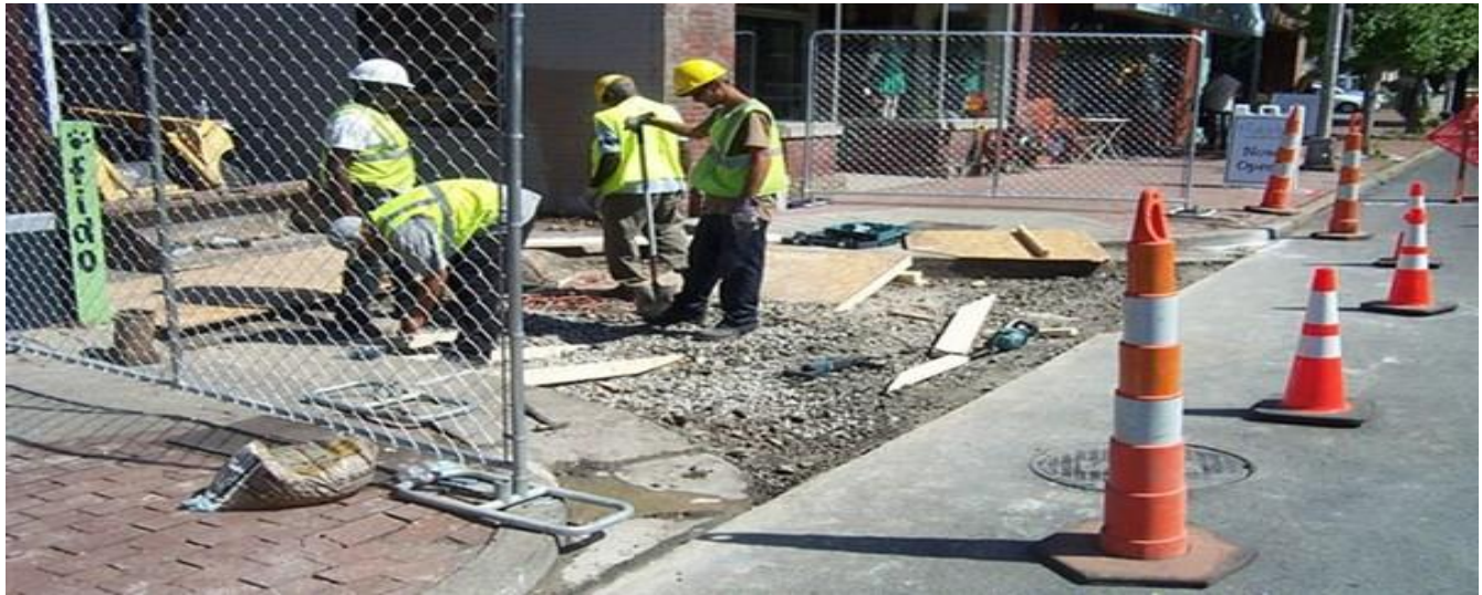
Intersection / Sidewalk Re-Construction – 21 st Avenue
