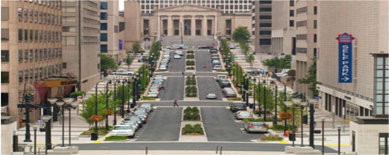
Deaderick Streetscape Improvement Project
