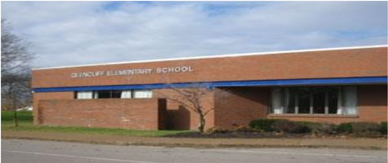
Glenclyff Elementary School
