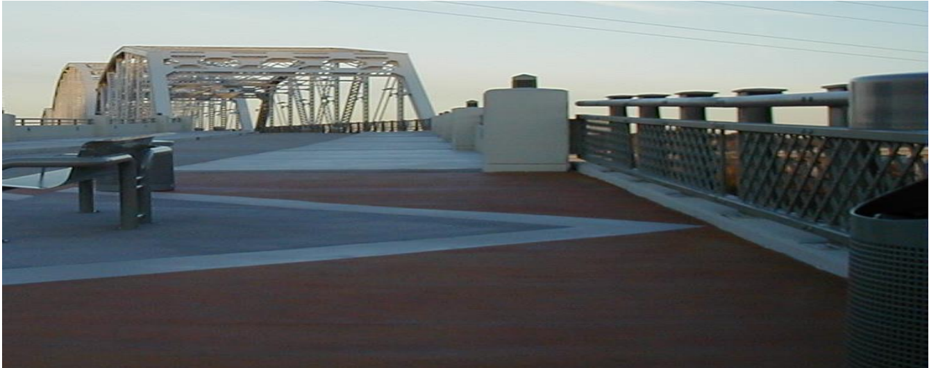
Shelby Street Bridge Walkway
