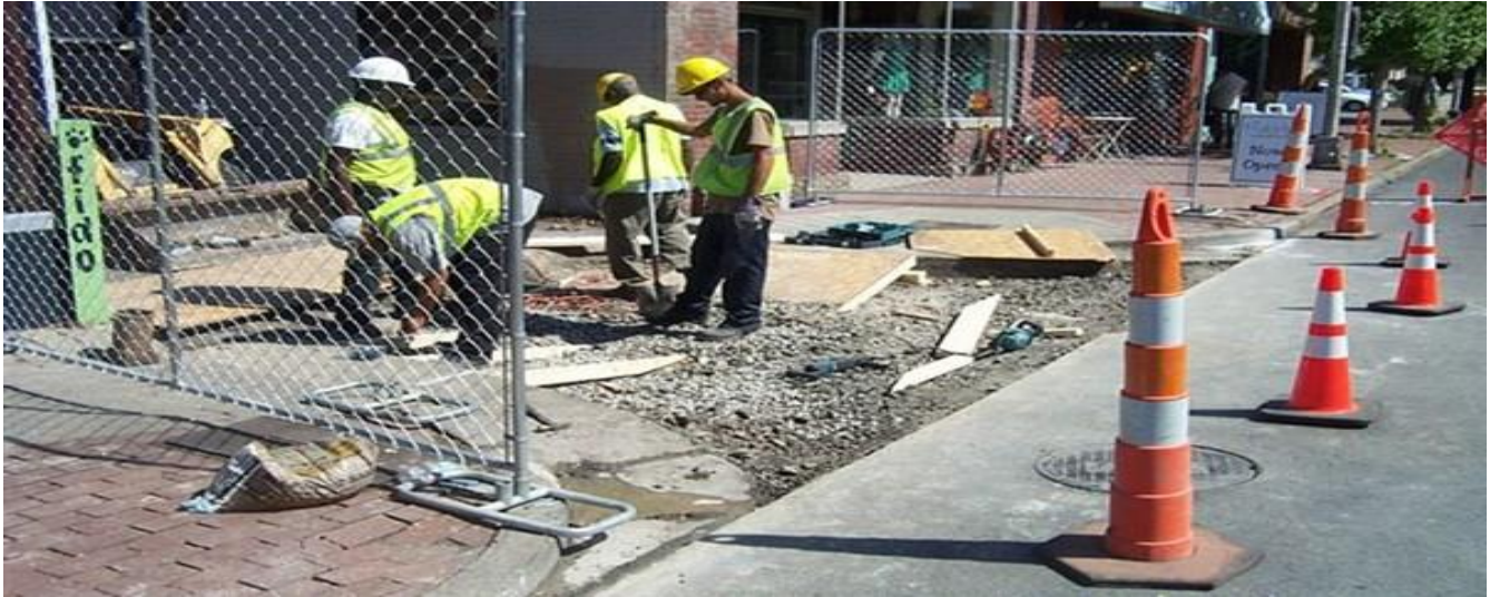
Intersection / Sidewalk Re-Construction – 21 st Avenue
