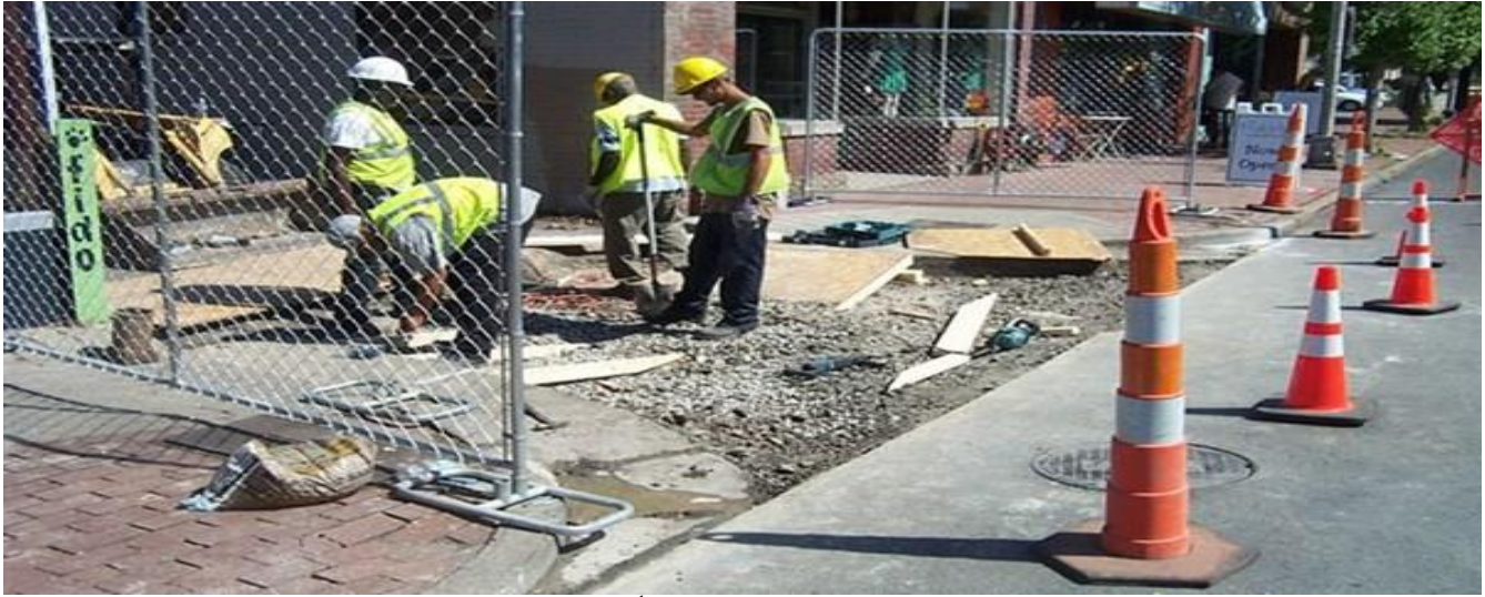
Intersection / Sidewalk Re-Construction – 21 st Avenue
