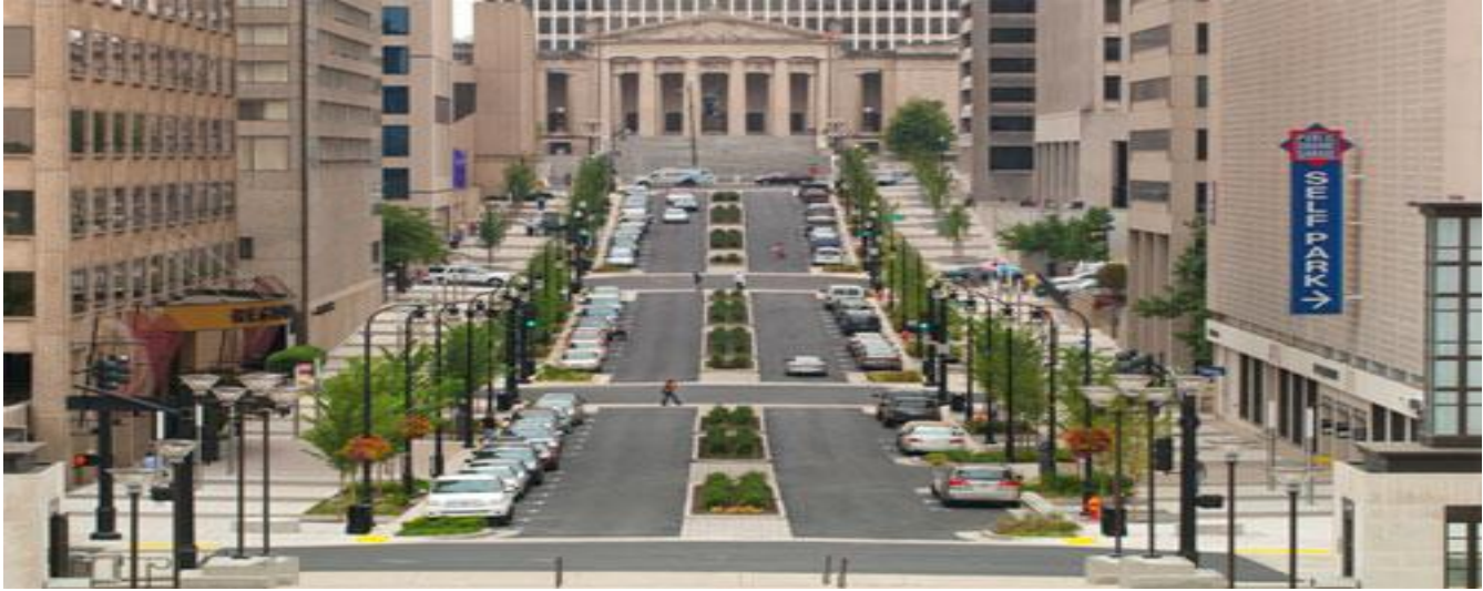
Deaderick Streetscape Improvement Project
