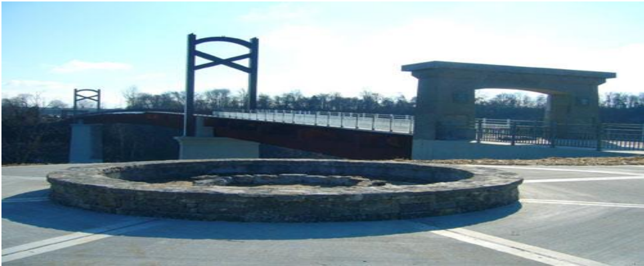
Cumberland River Pedestrian Bridge – Stones River Greenway
