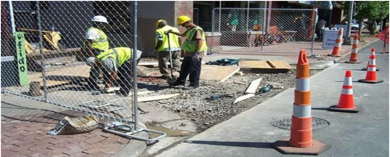
Intersection / Sidewalk Re-Construction – 21 st Avenue
