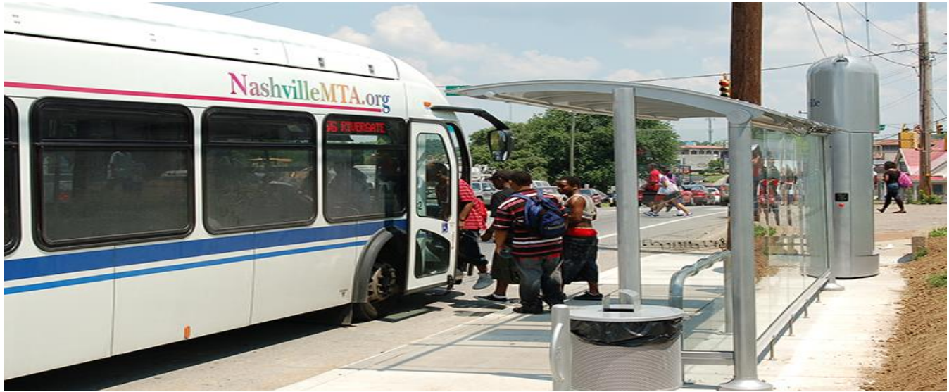
MTA's Bus Rapid Transit (BRT) Gallatin Road
