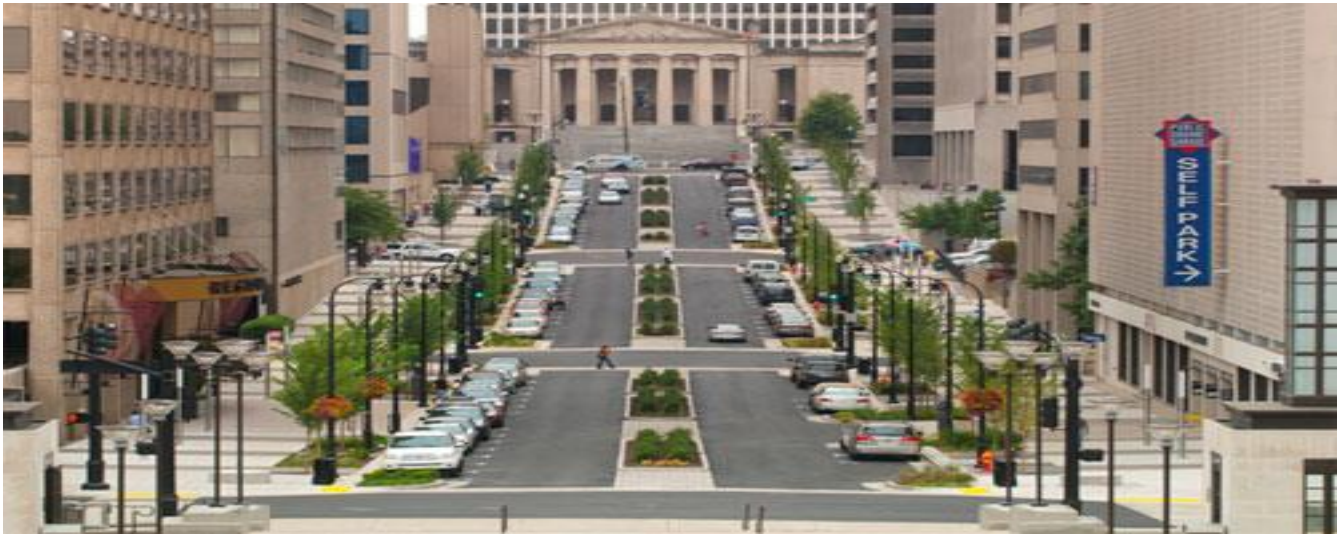
Deaderick Streetscape Improvement Project
