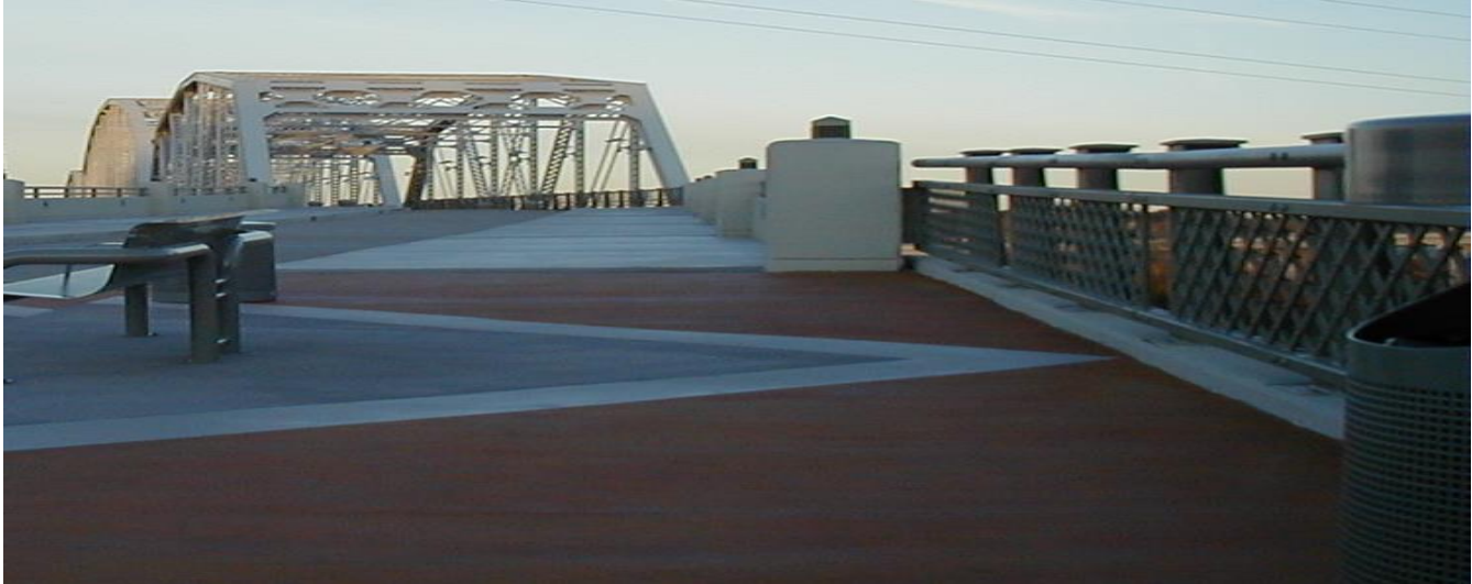
Shelby Street Bridge Walkway
