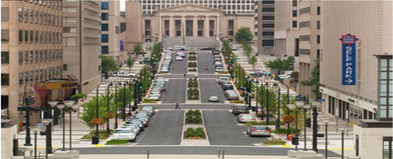
Deaderick Streetscape Improvement Project
