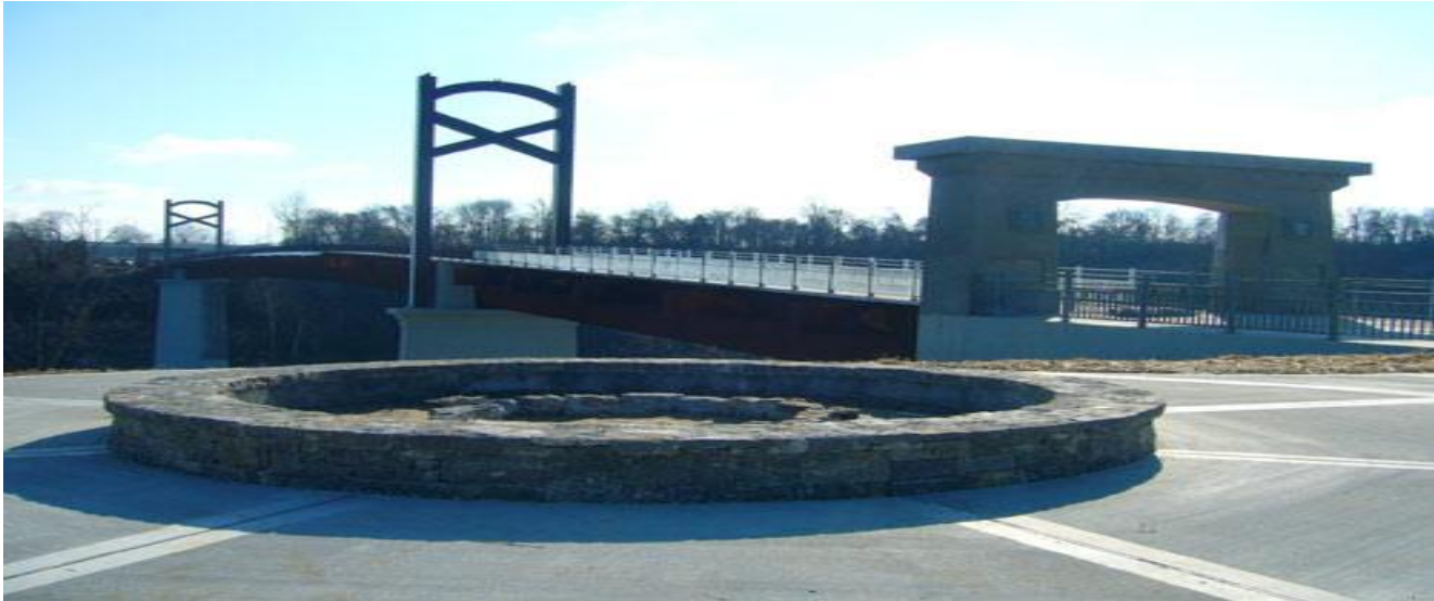
Cumberland River Pedestrian Bridge – Stones River Greenway
