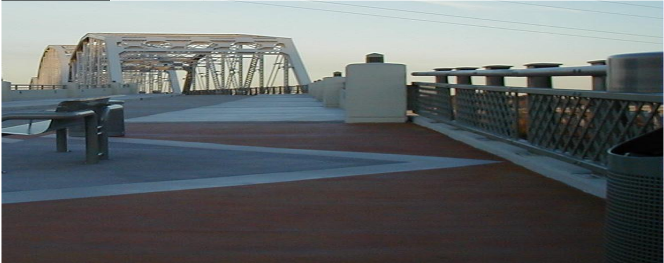
Shelby Street Bridge Walkway
