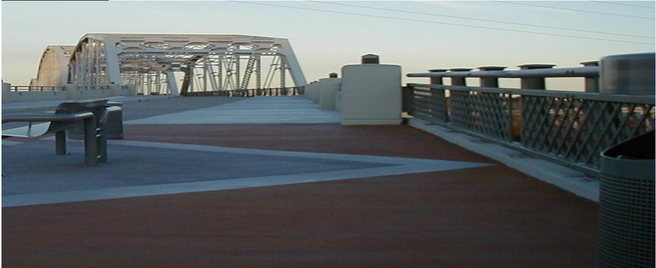
Shelby Street Bridge Walkway
