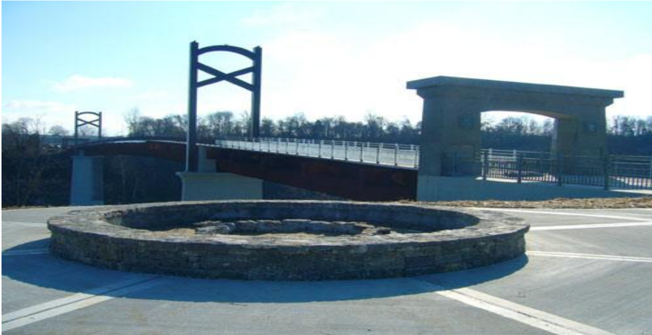
Cumberland River Pedestrian Bridge – Stones River Greenway
