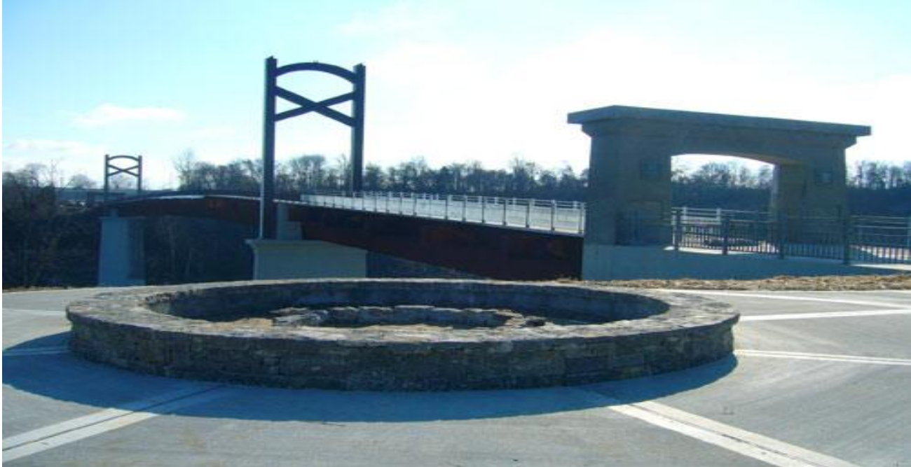
Cumberland River Pedestrian Bridge – Stones River Greenway
